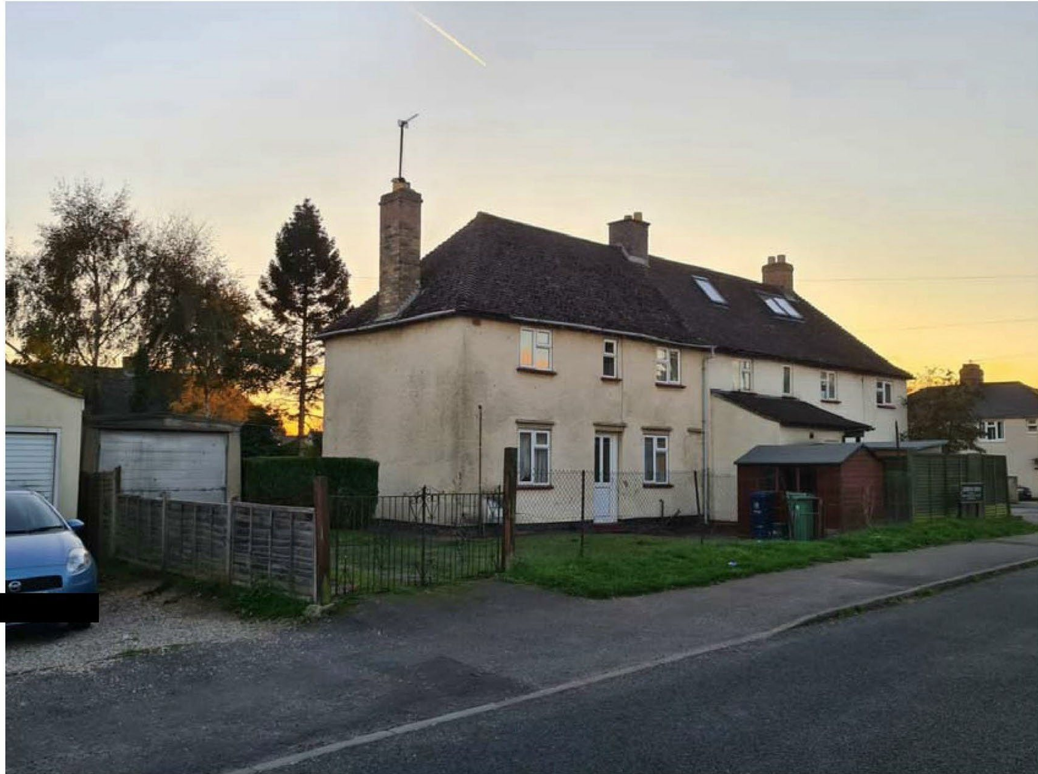
View of development plot from along Addison Drive.
