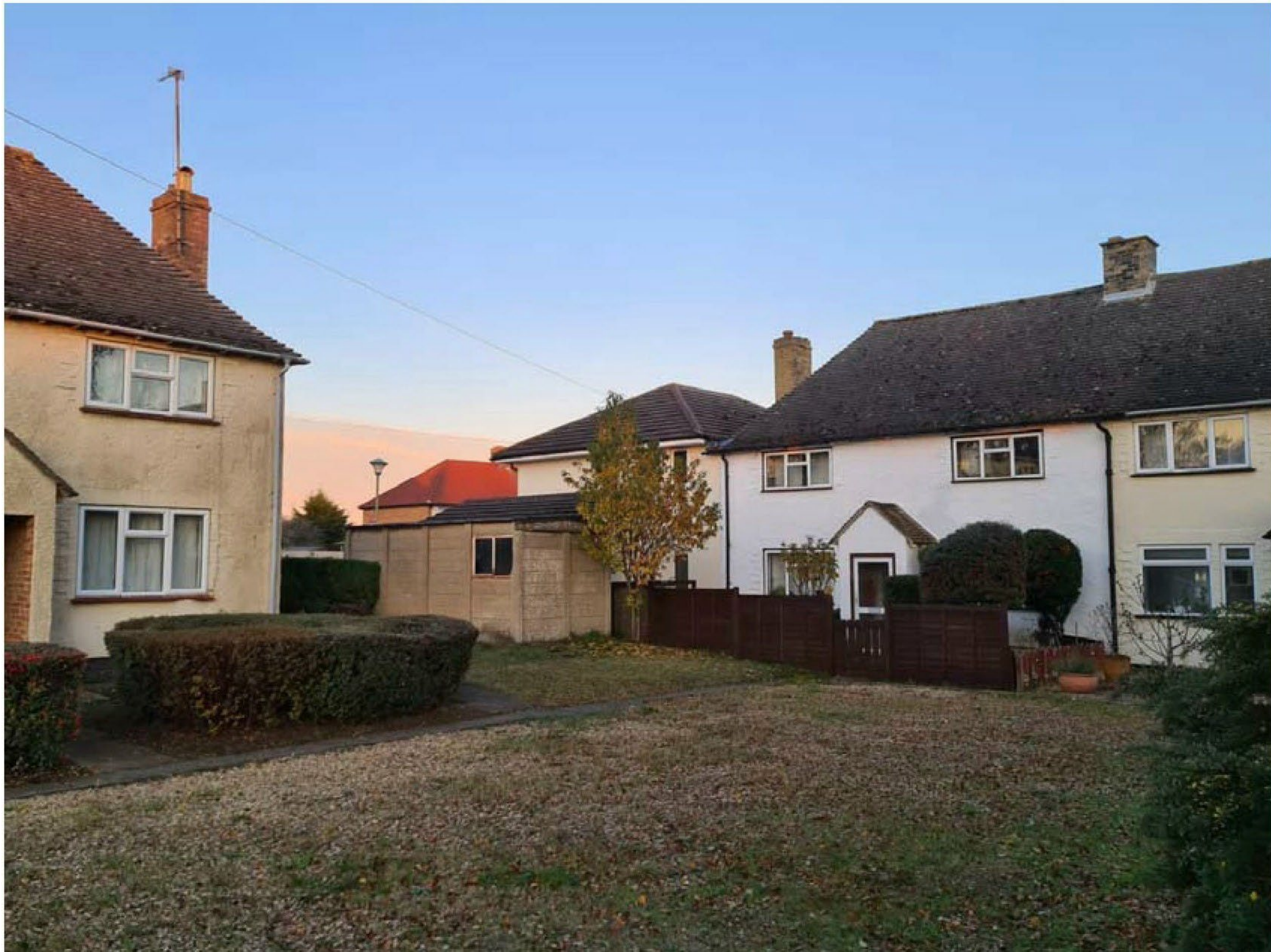
View of front of property with No. 116 to right and courtyard garden to front.
