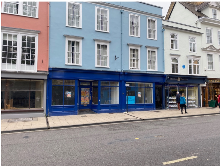
Photo A: Existing shop frontage
