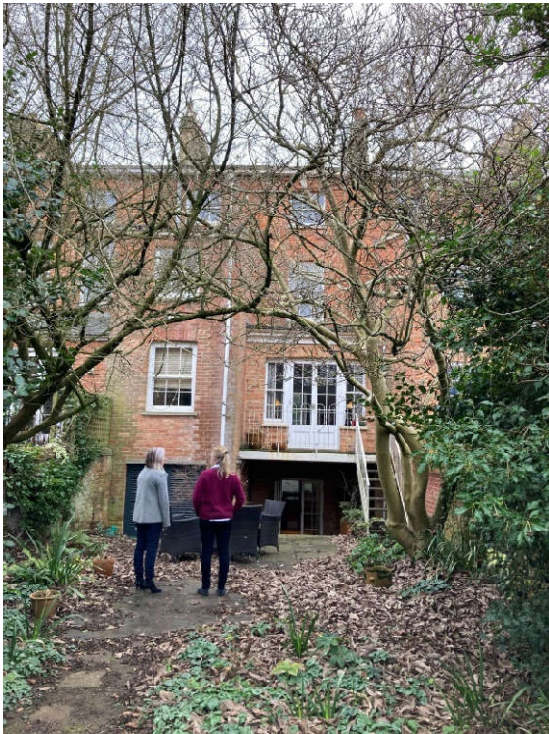
No.53. Rear elevation and garden
