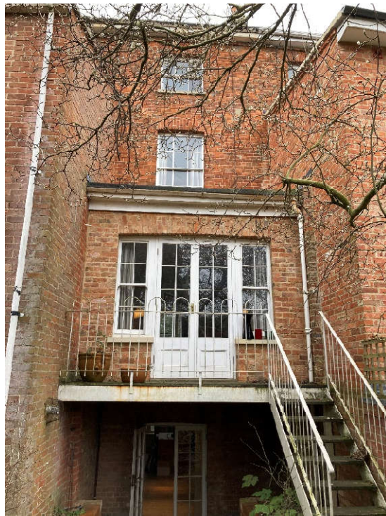
Existing infill extension
