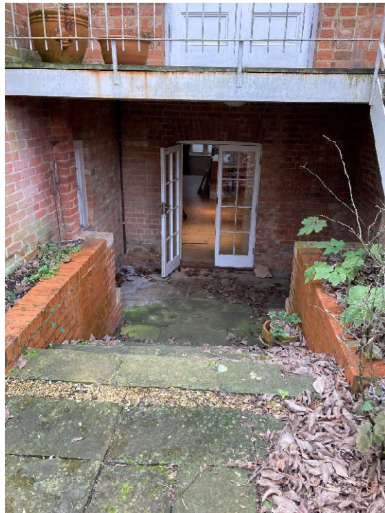
Existing rear undercroft and access
