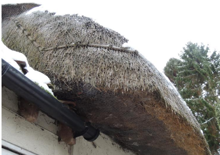
Photo 7: Showing mesh to western eaves
