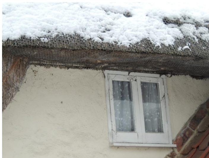
Photo 4: Northern gable. Note mesh
