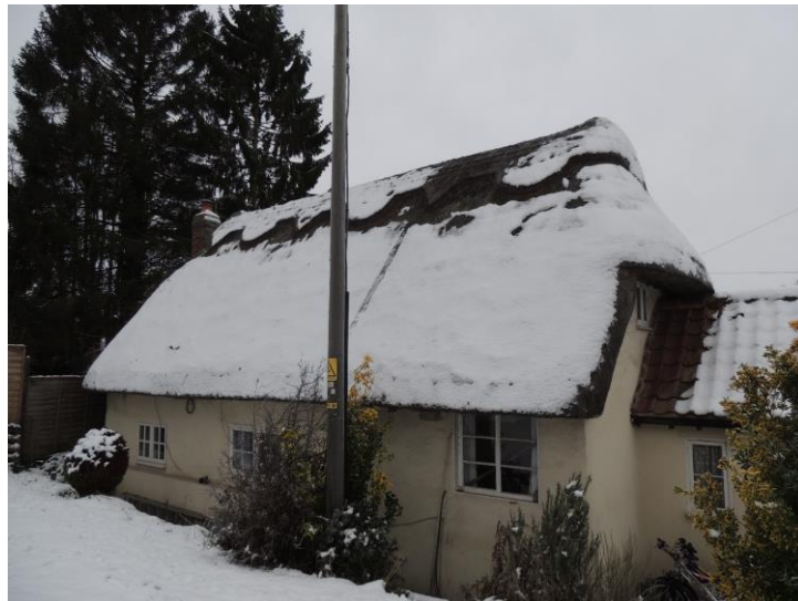
Photo 3: Northern and eastern elevations
