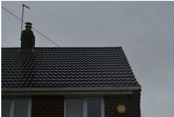
Figs. 3 & 4 External roof detail – no gaps/crevices present
