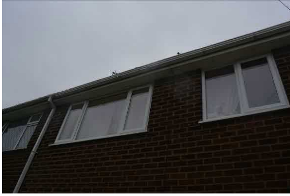
Figs. 5 & 6 UPVC Eaves fully sealed with no gaps/crevices present
