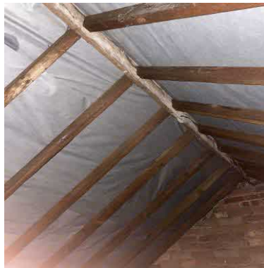
Figs. 8 & 9 Roof void lined with BRM
