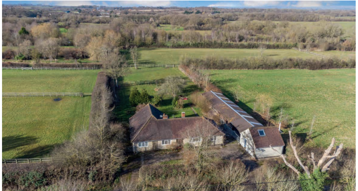
View of existing house, looking west
