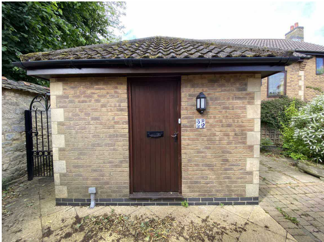
Above photos – existing front (east) elevation.
