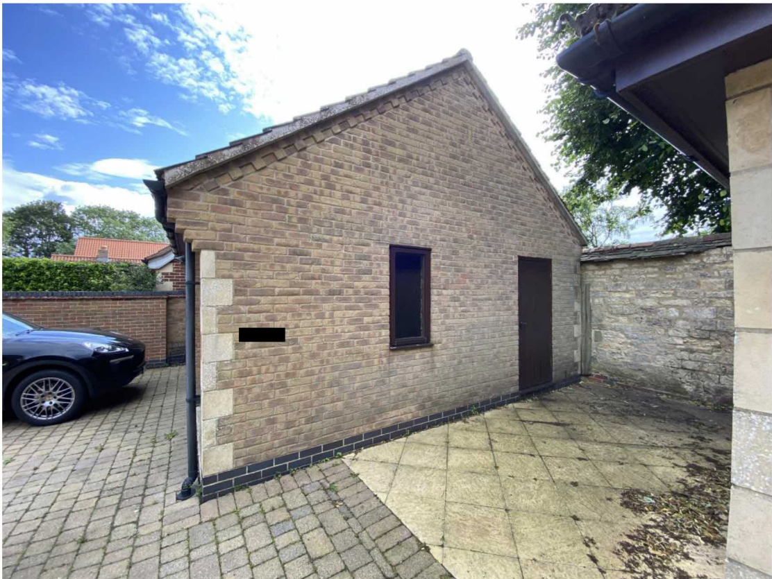
Above photos – existing detached garage and its relation to the property.
