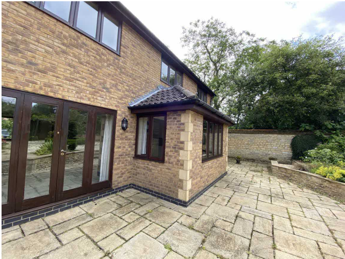
Above photos – existing rear (west) elevation.
