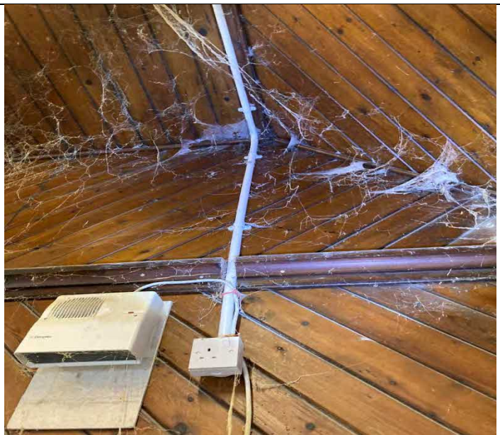
Photograph 3: Another view of the roof structure
