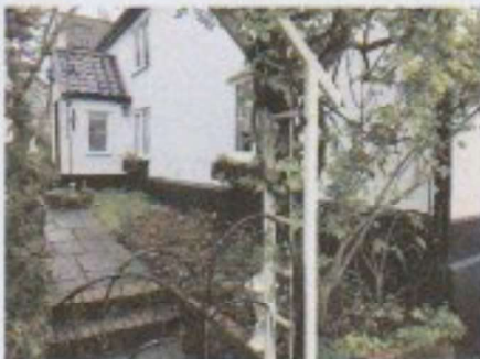
Photo 4: south elevation showing previous finish.
