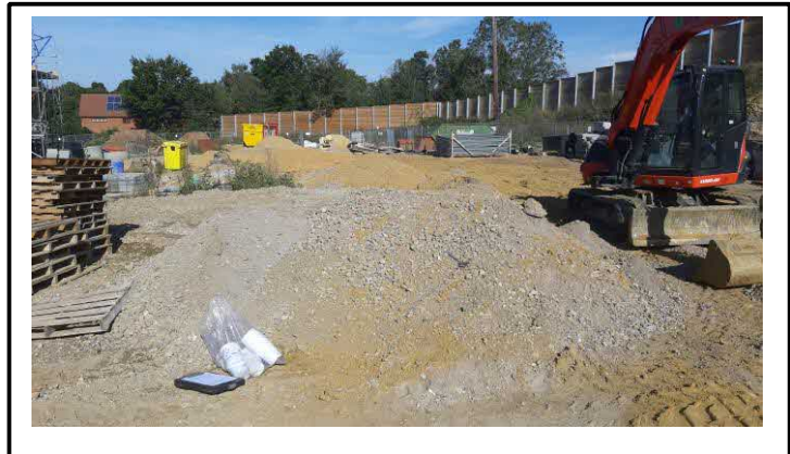
Type 1 Crush Stockpile – 10 October 2023
