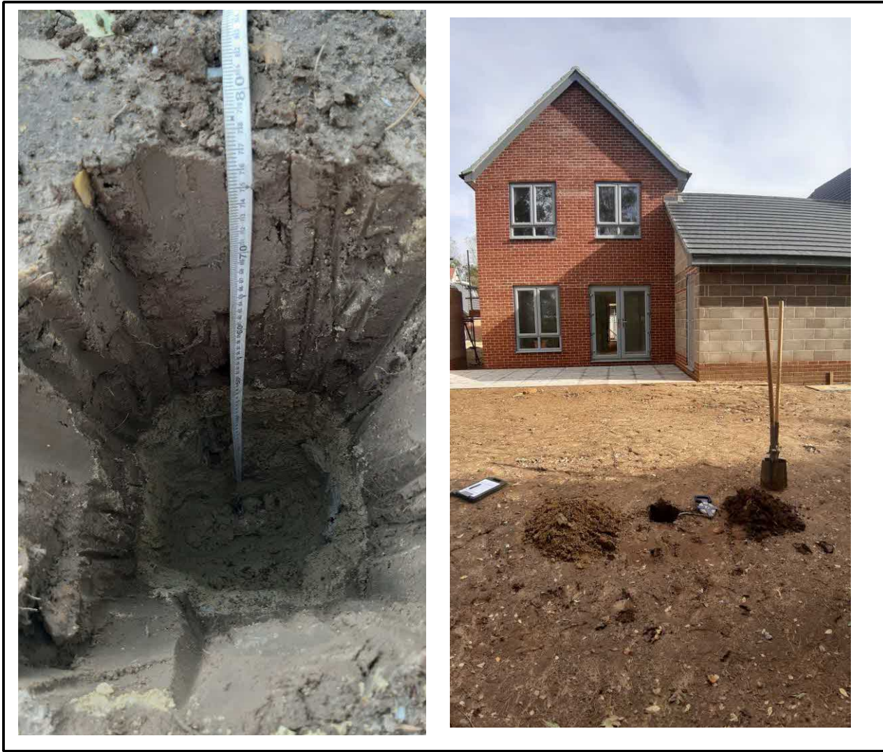
VA28 – Plot 31, 350 mm TS, 420 mm SS, Membrane
