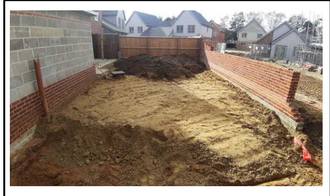
VA26 – Plot 24, Membrane placed at 820 mm below FFL, Partially Subsoiled/Topsoiled
