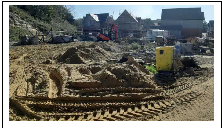
Subsoil Stockpile – 10 October 2023
