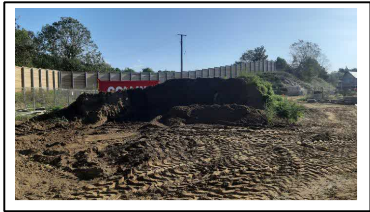
Topsoil Stockpile – 10 October 2023
