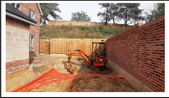
VA25 – Plot 22, Membrane placed at 700 mm below FFL
