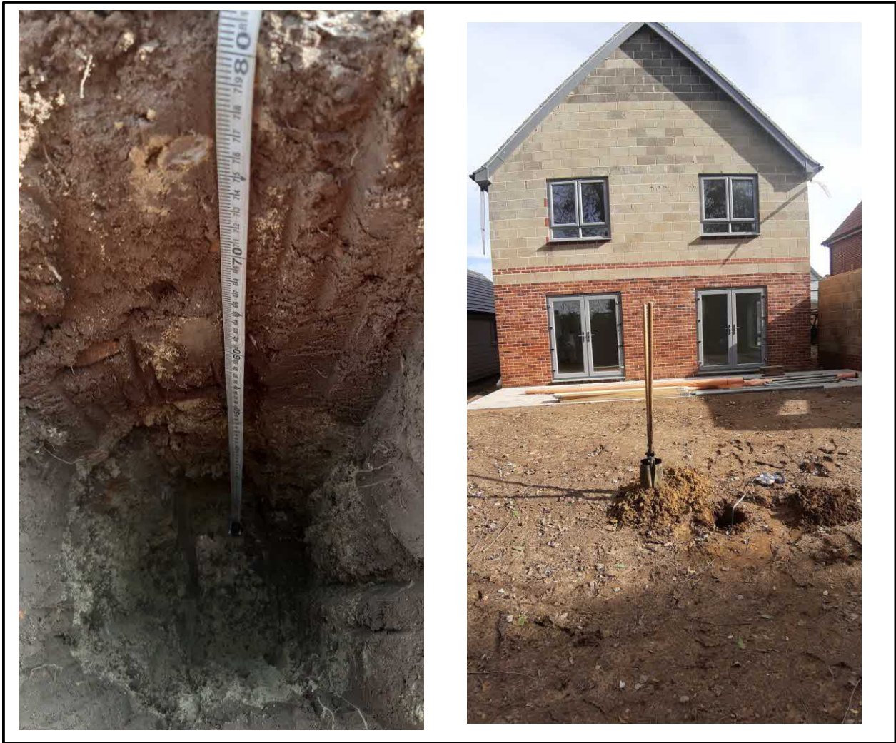
VA29 – Plot 32, 350 mm TS, 450 mm SS, Membrane
