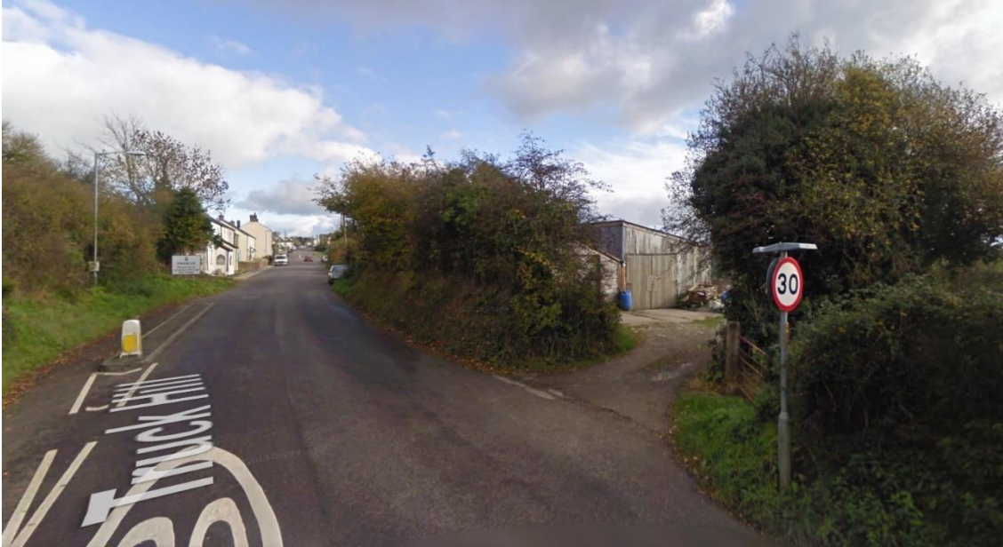
Fig 3: Image of access to existing site, Allotments and Pasture.
