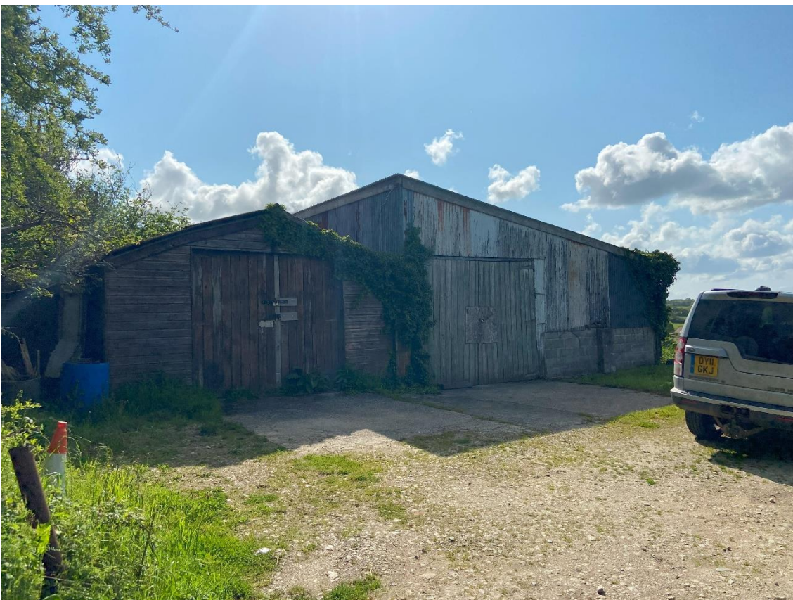
Fig 4: Existing structures and hardstanding.
