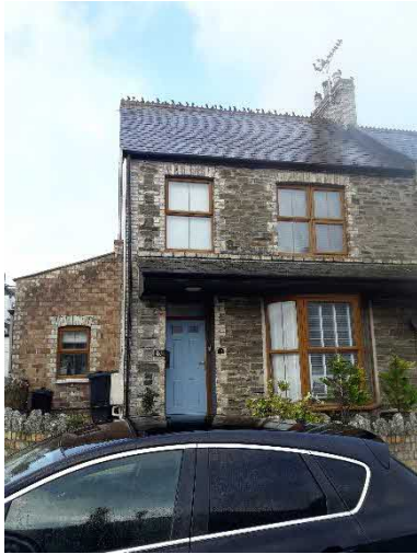
Figure 1 East side of the building
