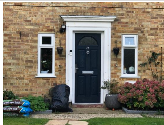
Photograph 8: The uPVC front door and wooden surround at the property where the proposed porch will be constructed. No PRFs noted.
