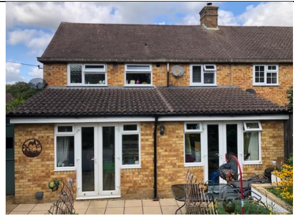
Photograph 2: Rear elevation and part of the back garden of the property.
