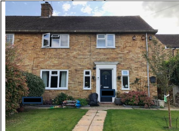
Photograph 1: The front elevation and part of the front garden of the property.
