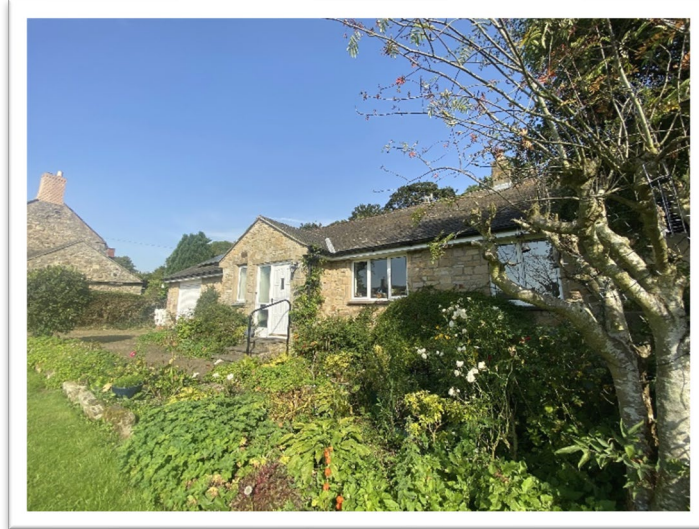
Figure 13 West elevation of Braeside
