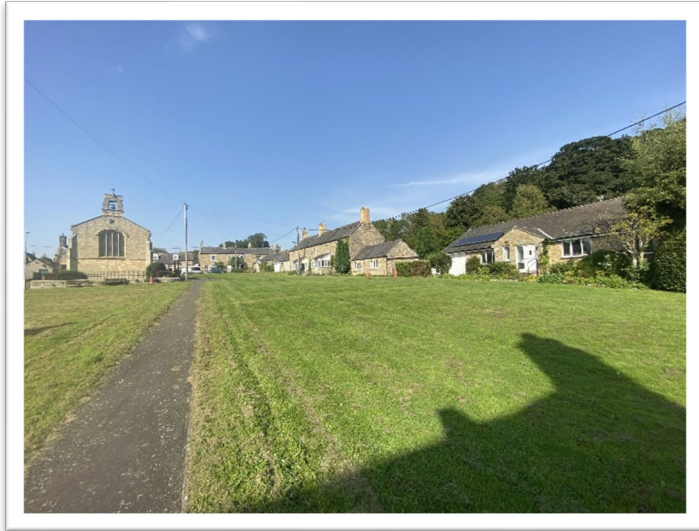
Figure 12 Looking northwards from Town Farm with Braeside to the right and the Church of St George to the centre left
