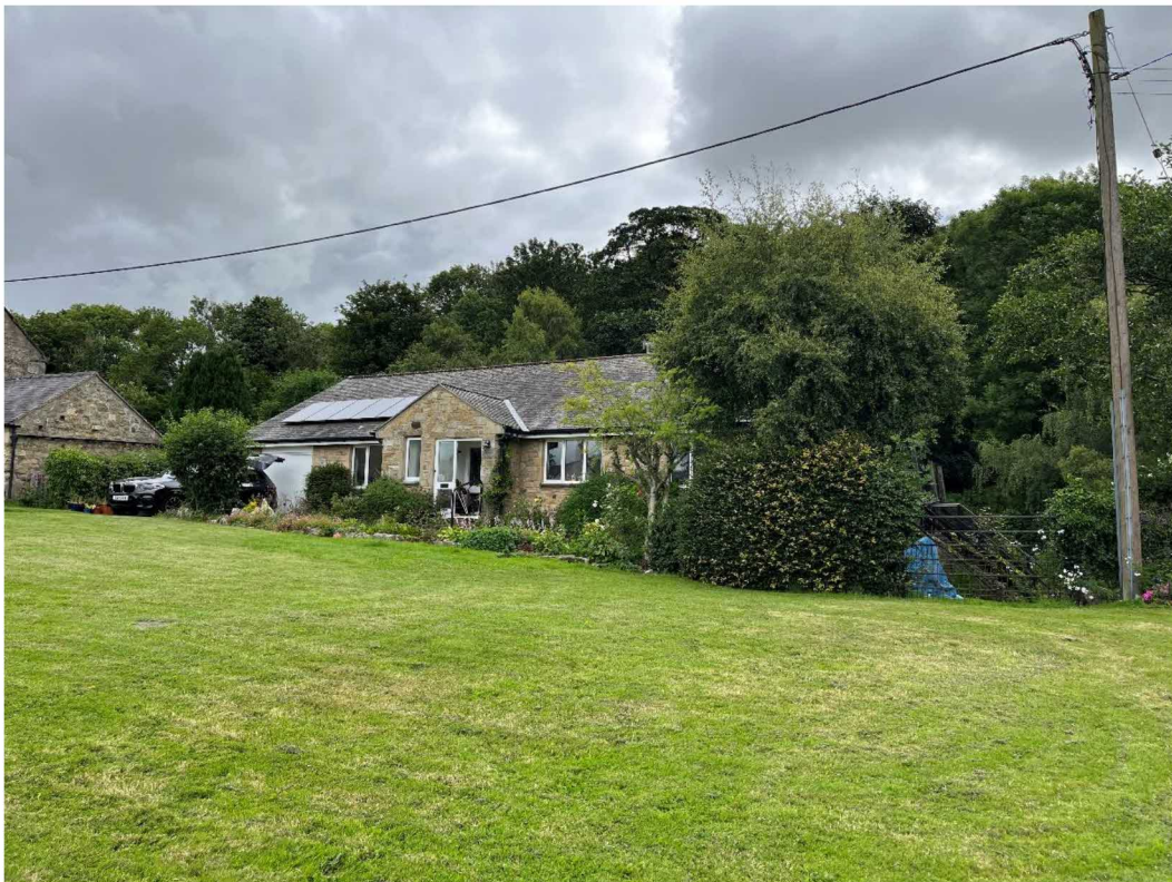
Property fronting The Green, reasonable mature screening to be retained
