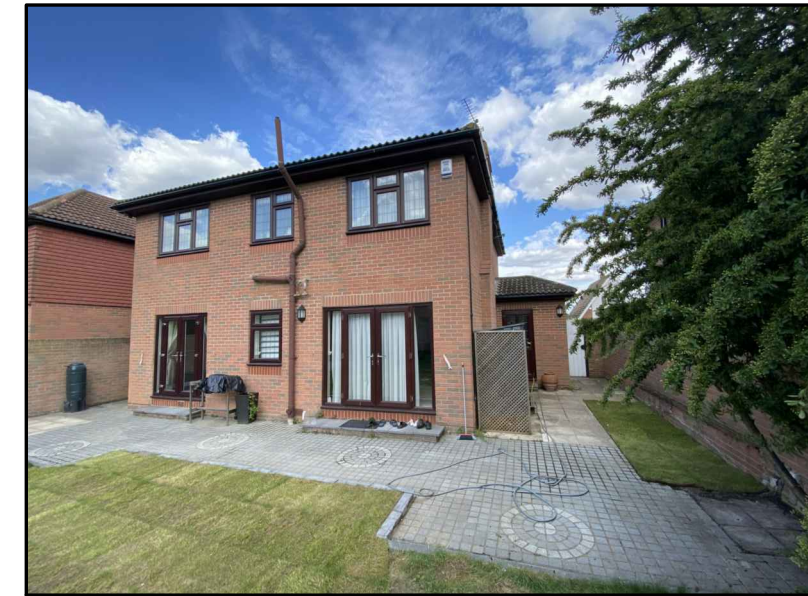
EXISTING REAR & SIDE VIEW
