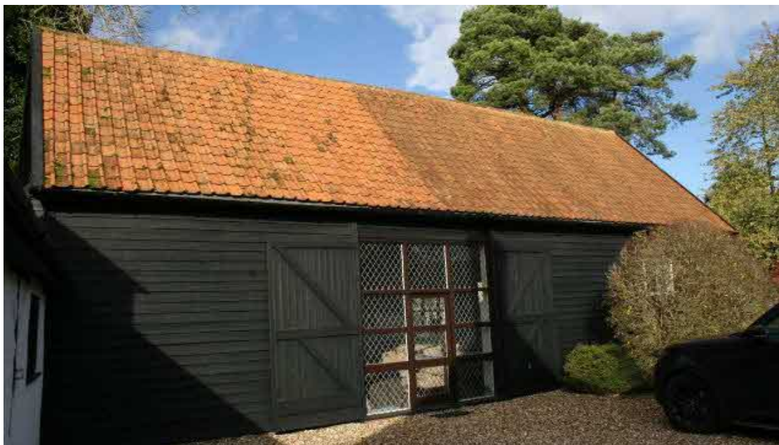
The south elevation of the Listed Barn.
