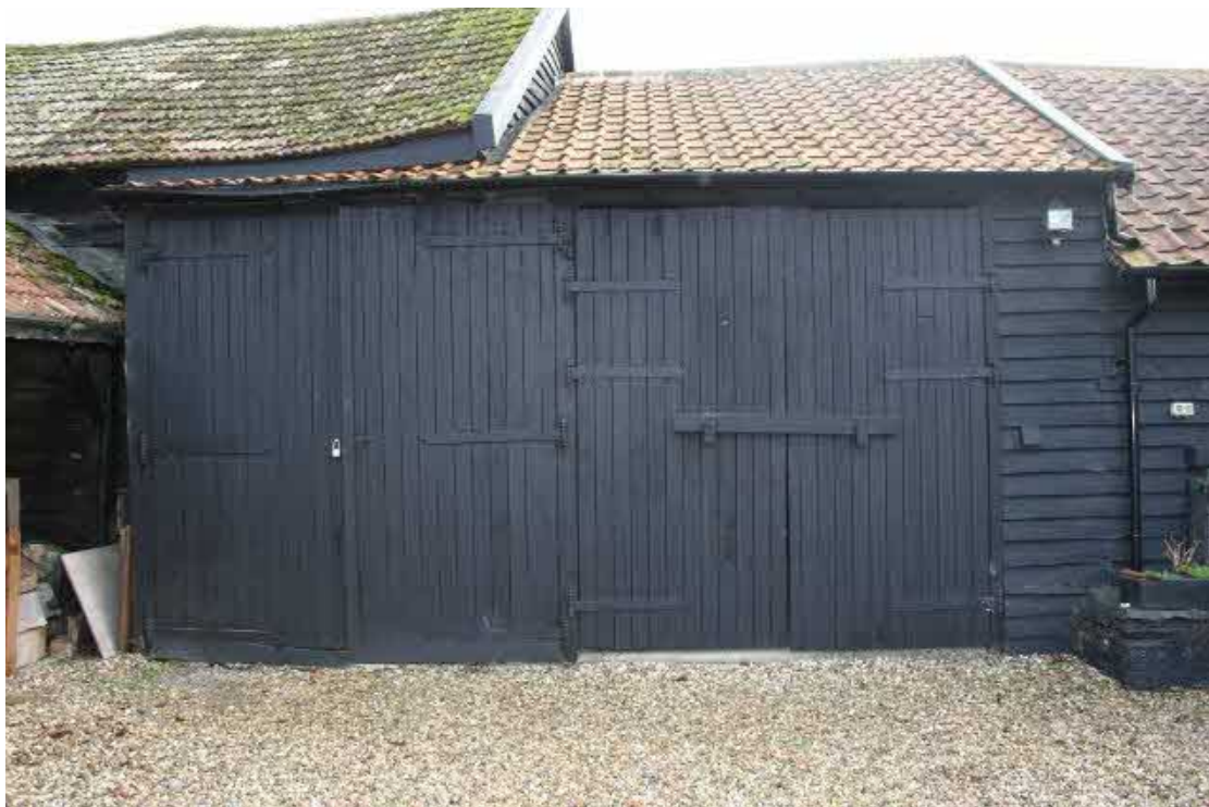
The north elevation of the Workshop with garage doors.
