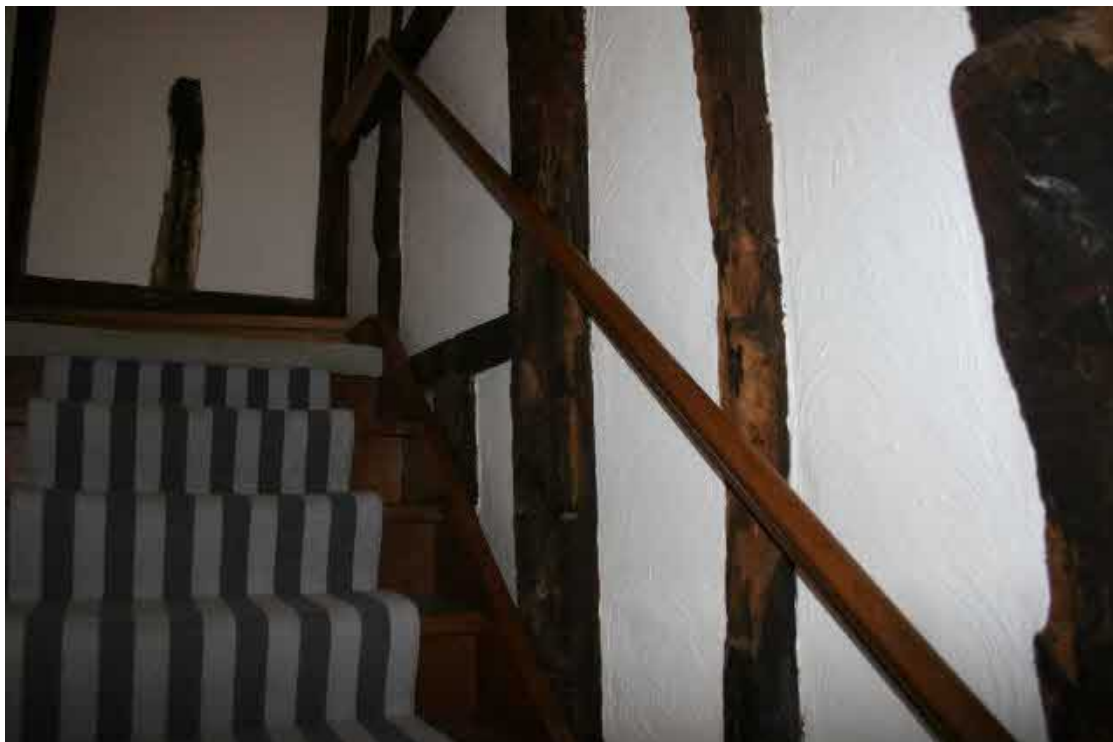
The frame exposed in the stairwell in the west wall.
