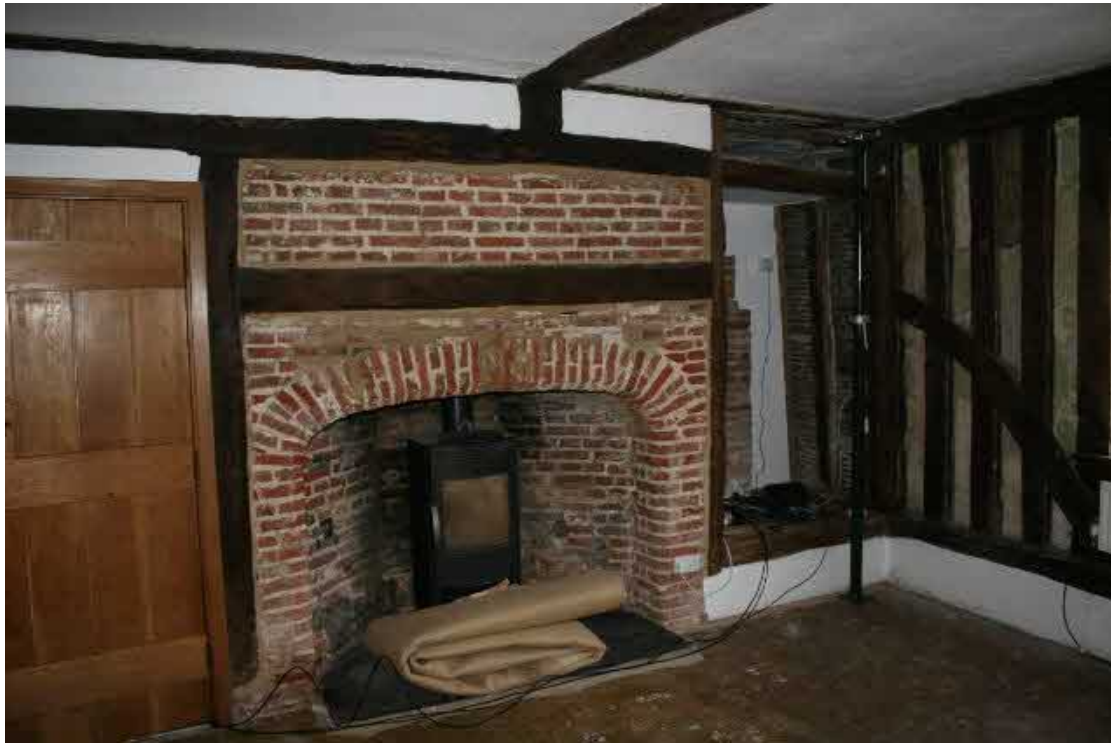
The fireplace in the north wall. Looking NE.
