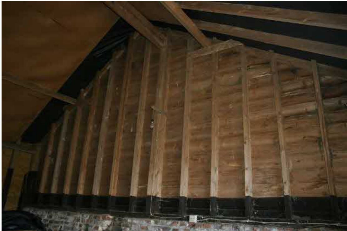
LC20th studwork in the west wall of the Garage.
