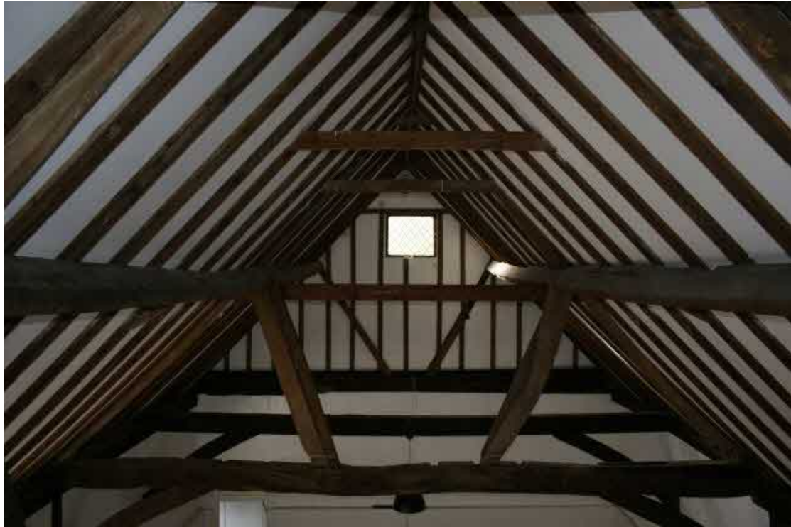
Looking W across the tie-beams.
