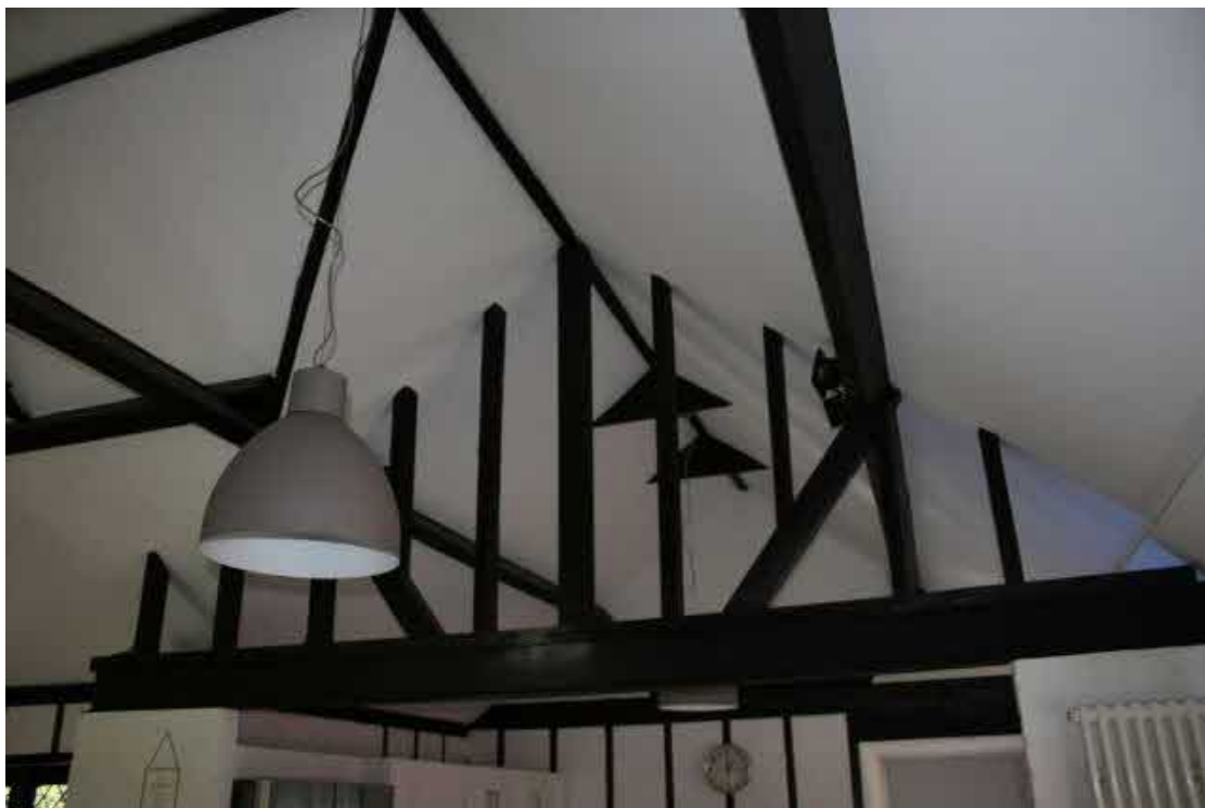
The central truss over the Kitchen.
