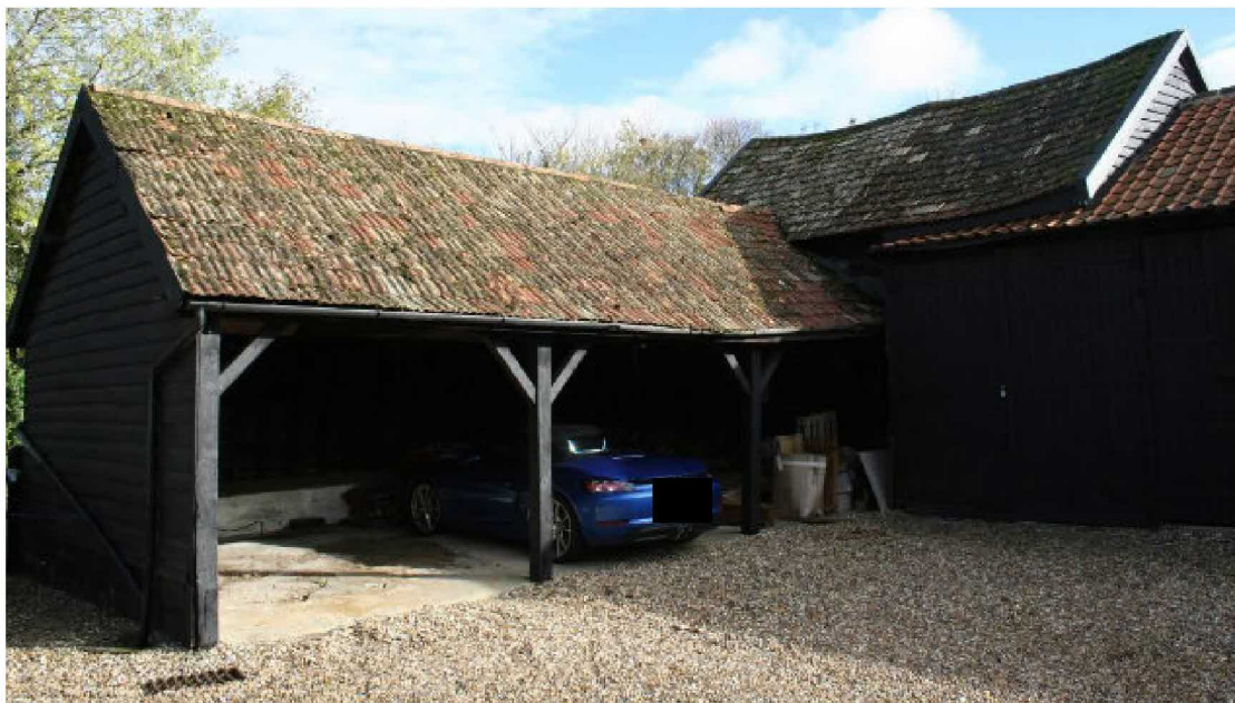
The west elevation of the Cart Lodge.
