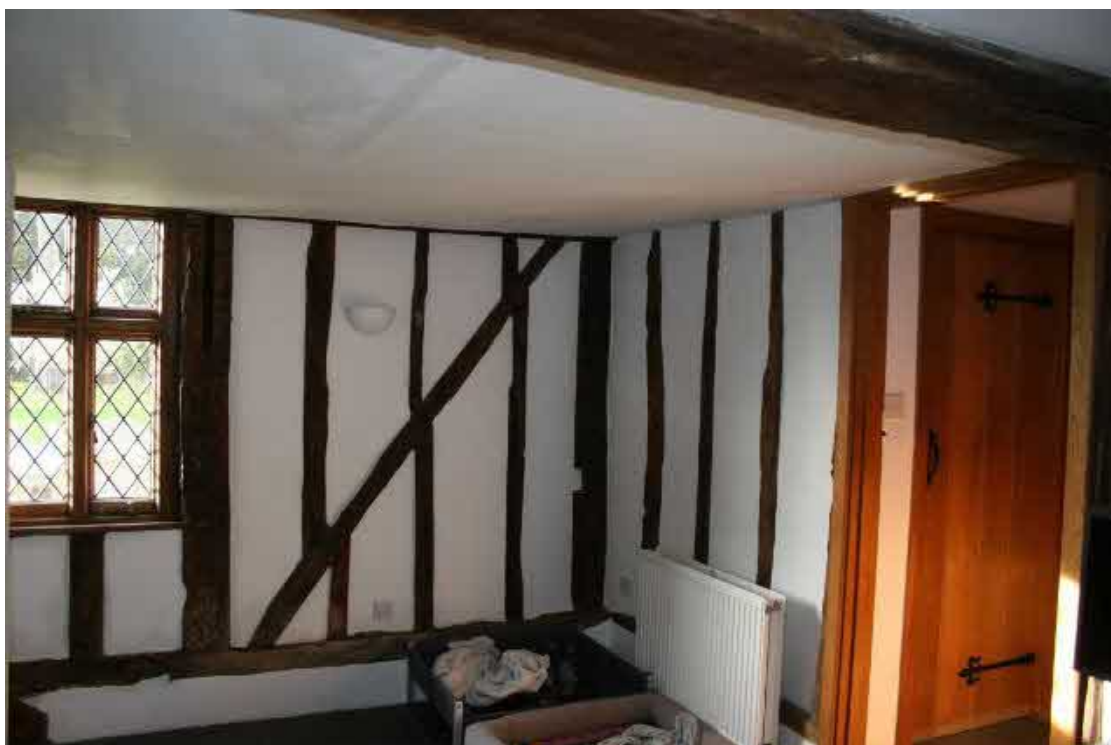
Looking NW in the Entrance Hall.
