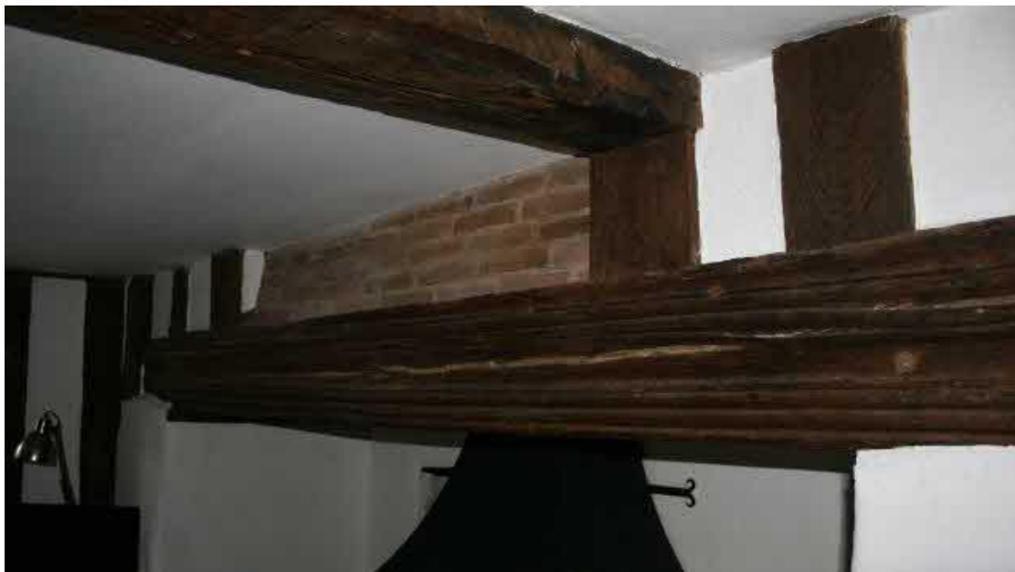
Detail of the roll moulded bressummer in the fireplace.
