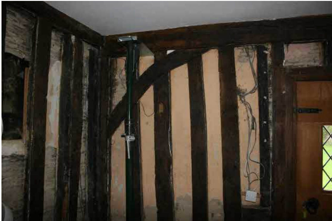
Detail of the curved brace in the SW corner.
