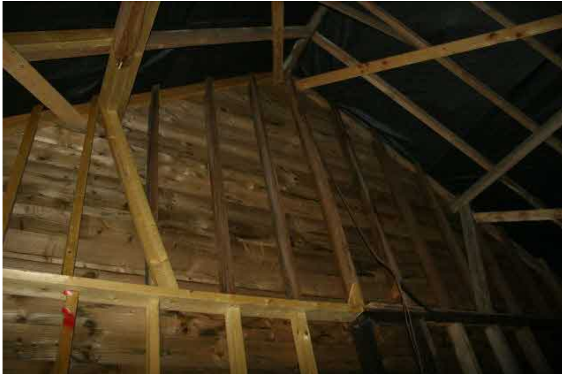
The west wall has been largely replaced in the LC20th.
