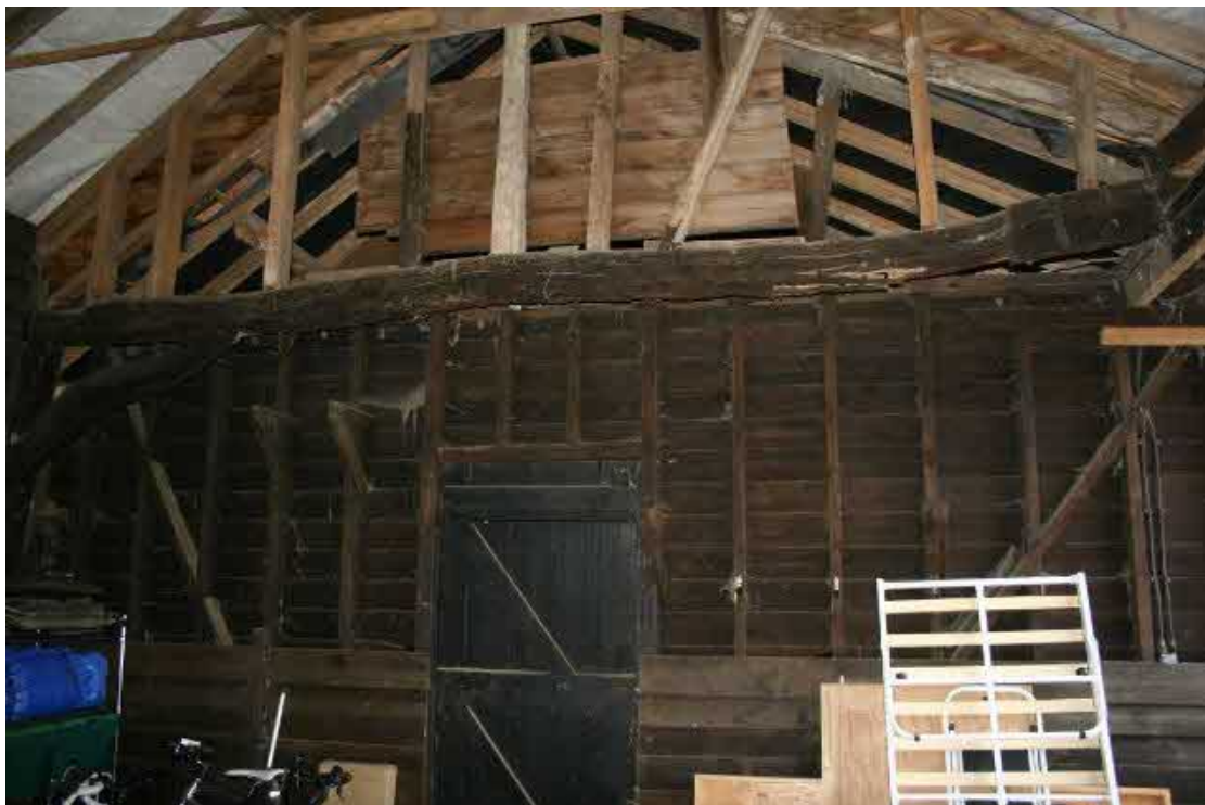
The west wall of the Workshop seen from inside looking W.
