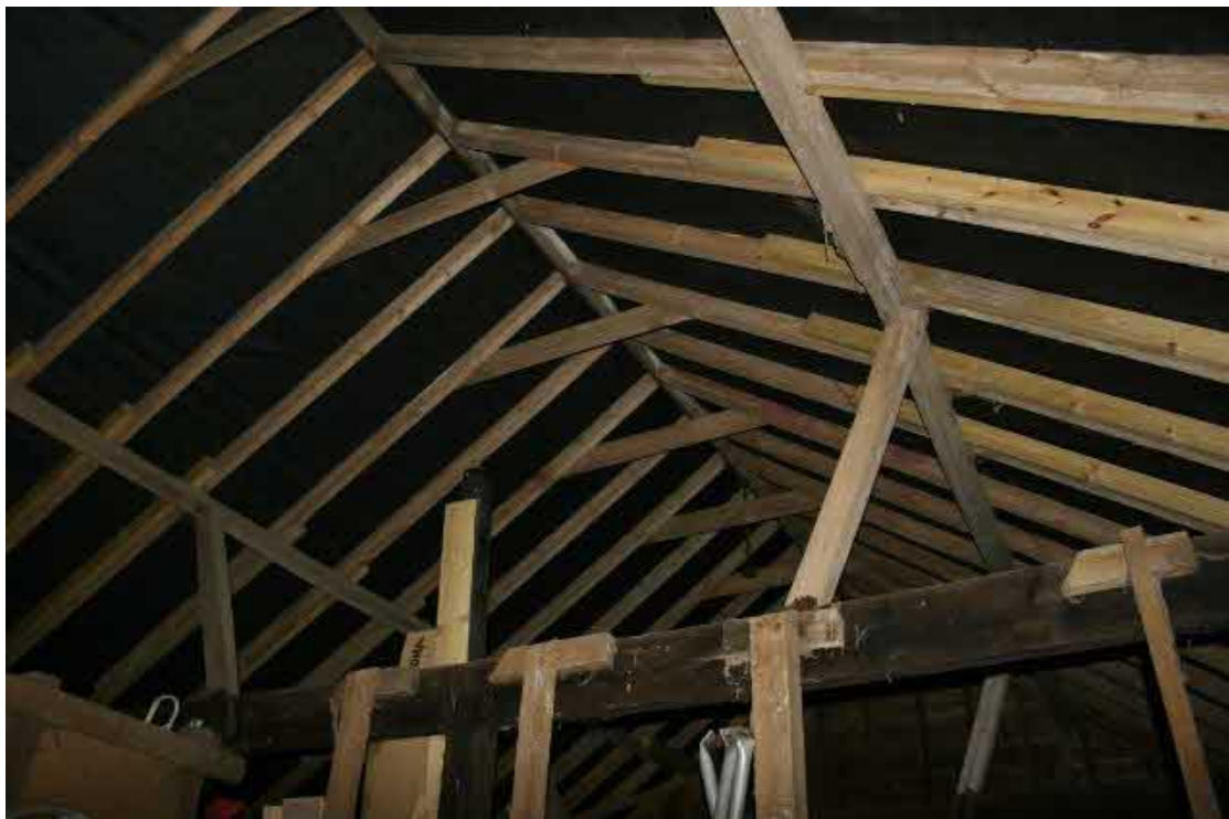
The roof structure above the loose box and stalls looking W.
