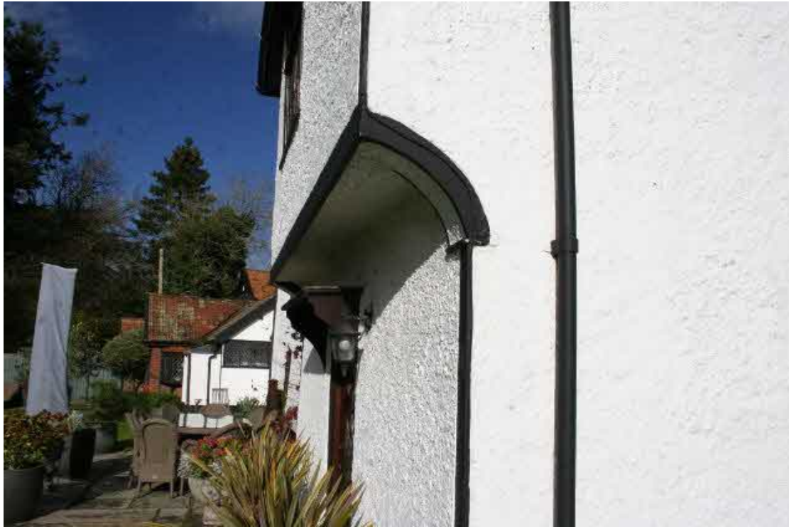
Detail of the render and the jetty brackets.
