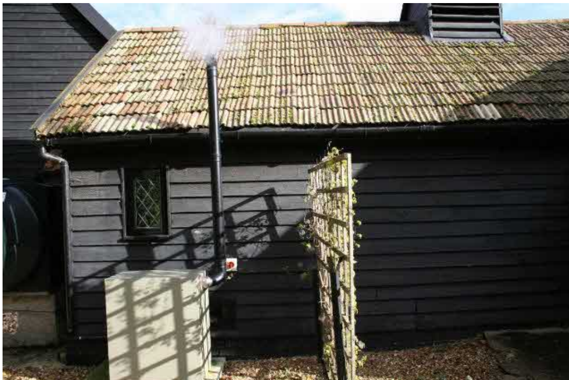
Weather-boarded section of the west elevation of the Kitchen.
