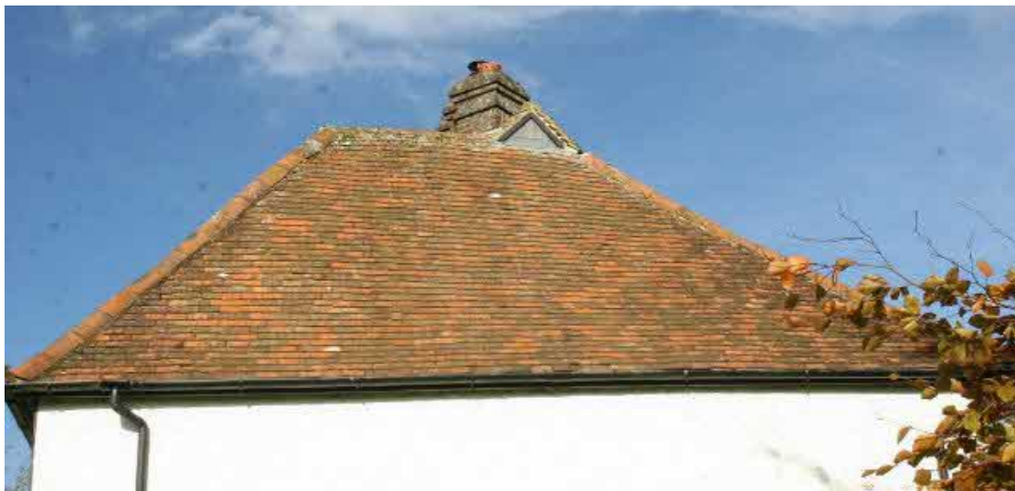
Detail of the roofline above the cross-wing.
