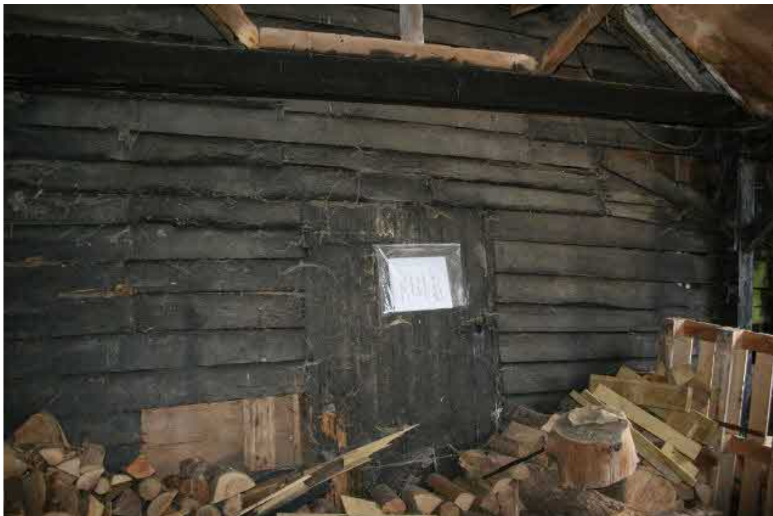
The pedestrian doorway into the Workshop.
