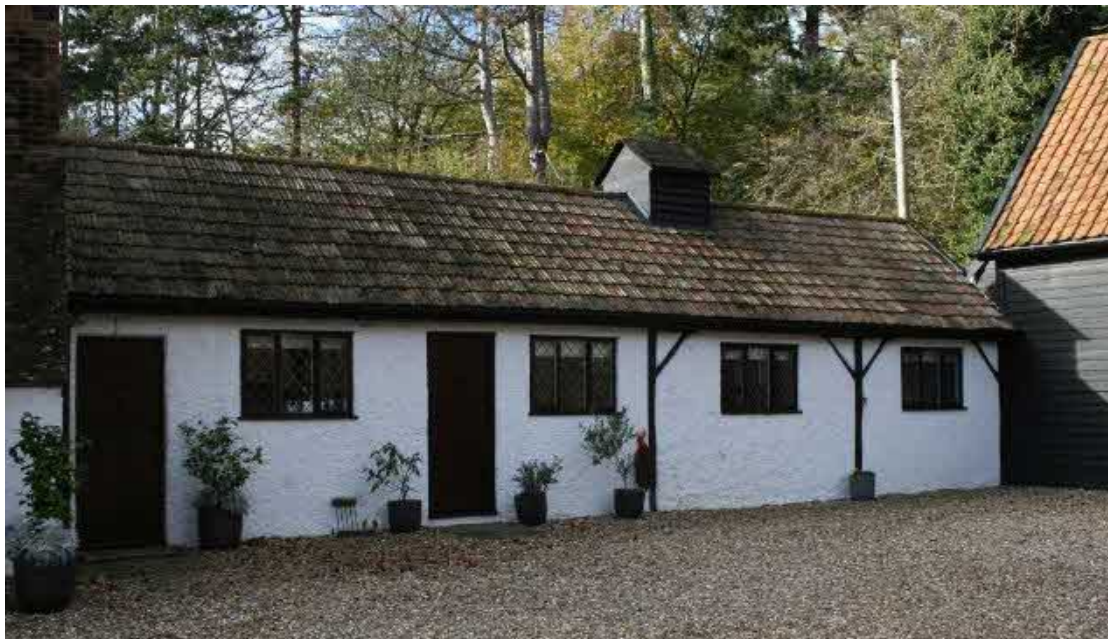
The eastern elevation dates to the LC20th.
