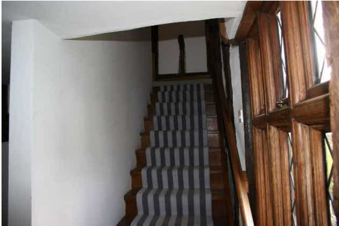
C20th staircase up to the first floor.
