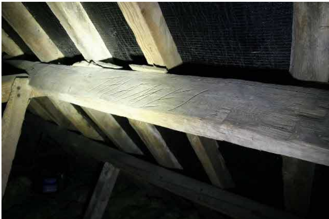
Side purlin with bracking mark 'Thames'.
