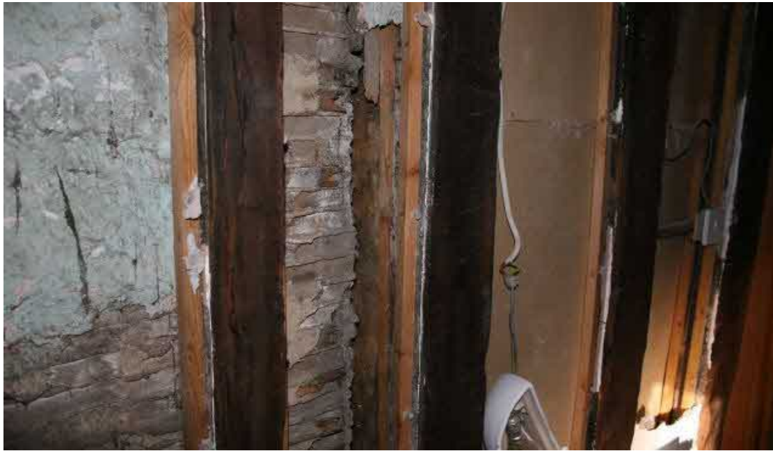
Detail of the lath and daub and LC20th plasterboard.
