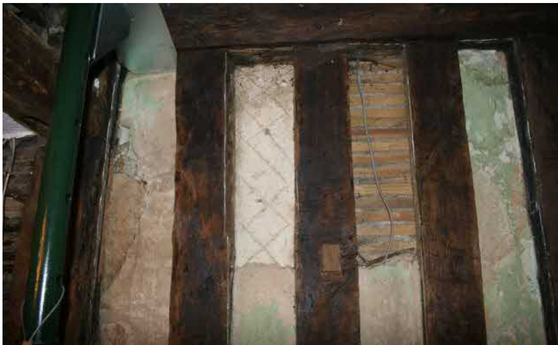
Lath and daub finish on the east wall.
