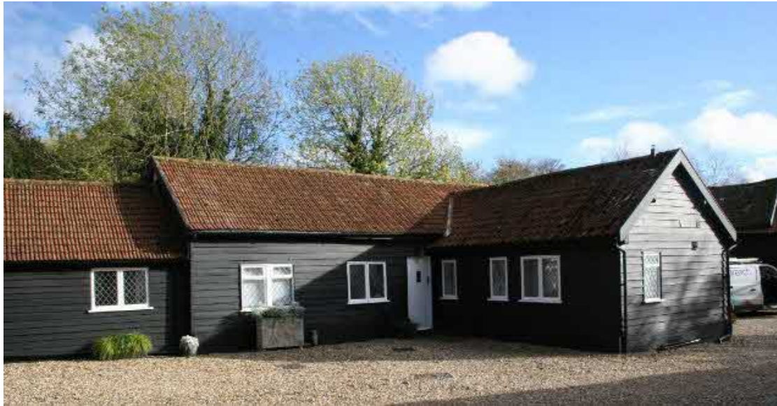
The north and west elevations of the Co age.
