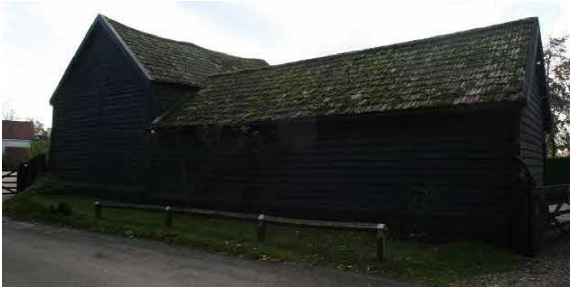
The east elevation of the Cart Lodge and the Workshop.
