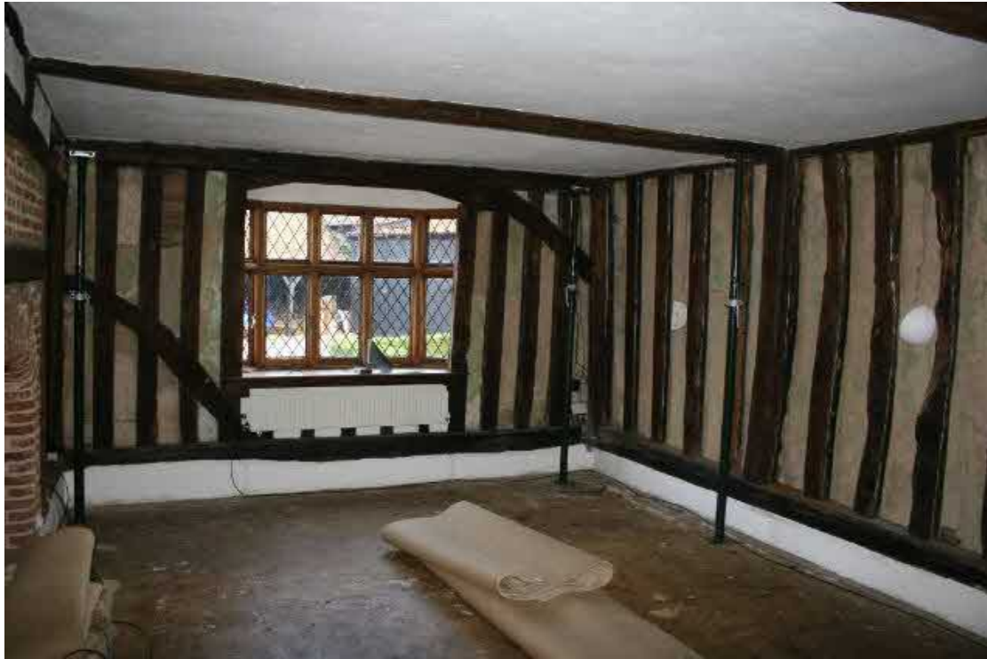
Looking E in the Cross-wing. Note the asymmetric braces.
