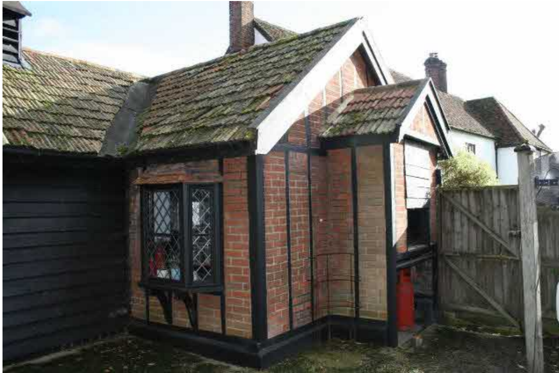
The kitchen extension and boiler house. Looking SE.
