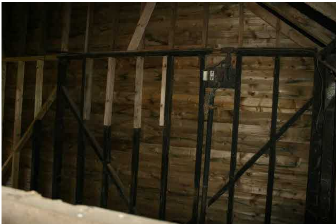
Sections of older C20th framing have been conserved.
