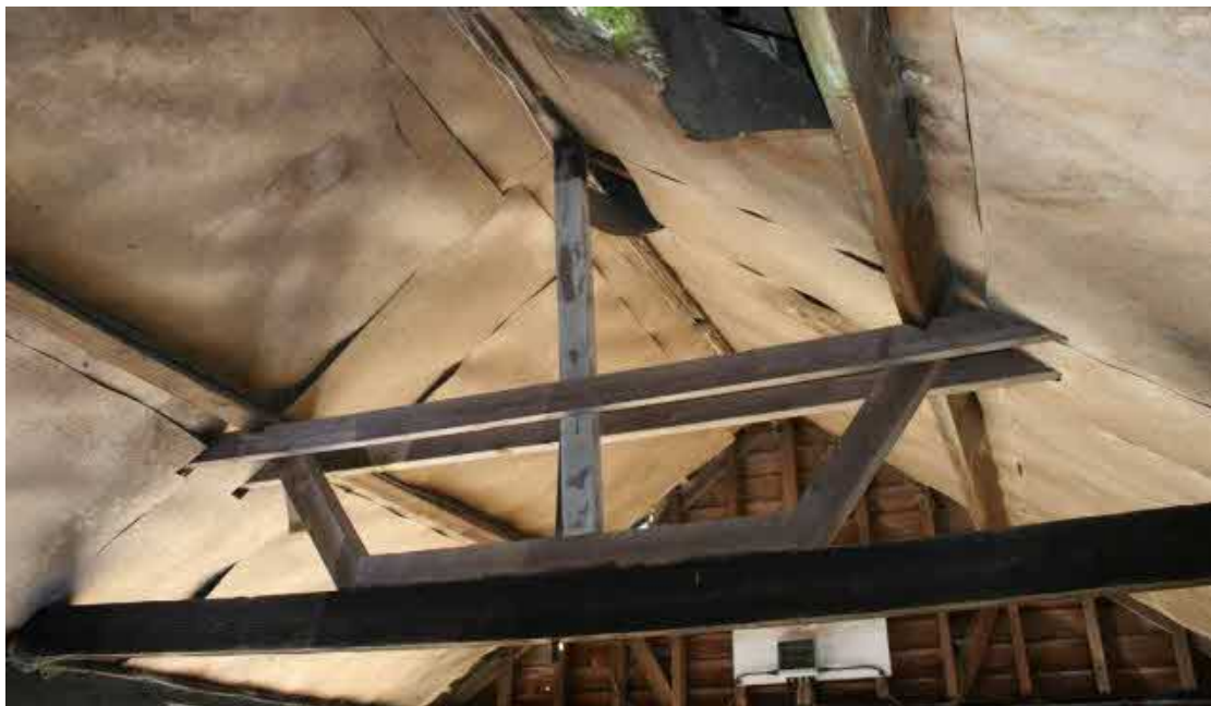
Looking N in the roof structure.
