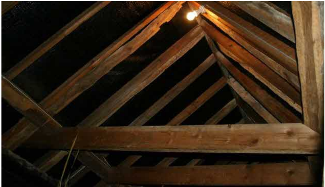
Detail of the roof over the main range. Looking N.
