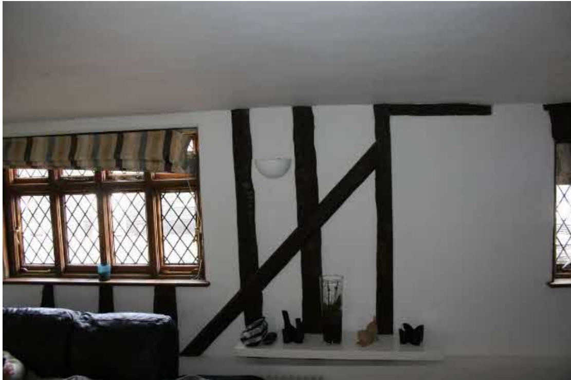
Fake LC20th frame in the east wall and earlier doorframe.
