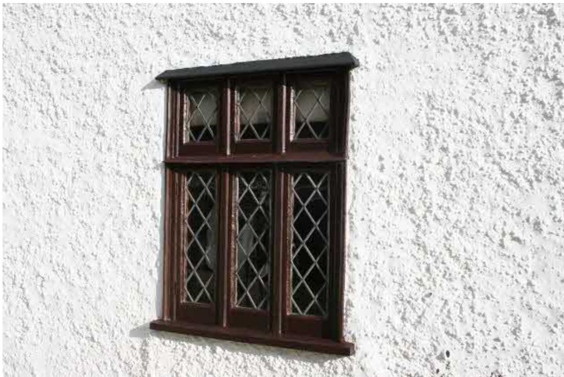
Detail of one of the ground floor windows.
