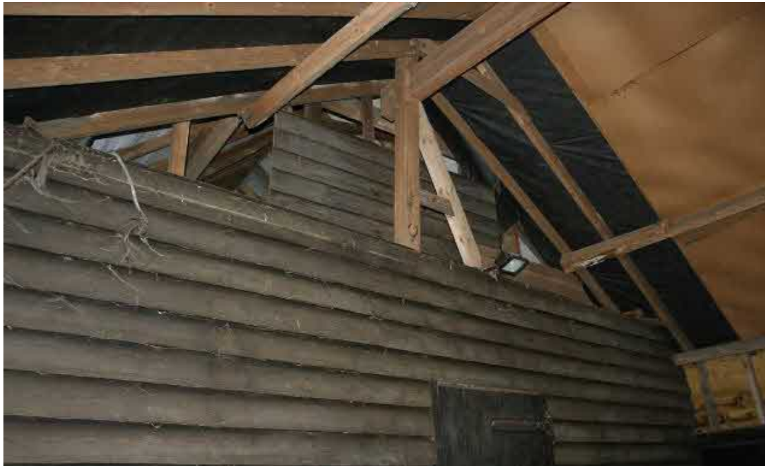
The C20th cladding of the Workshop in the west wall seen in the Garage.
