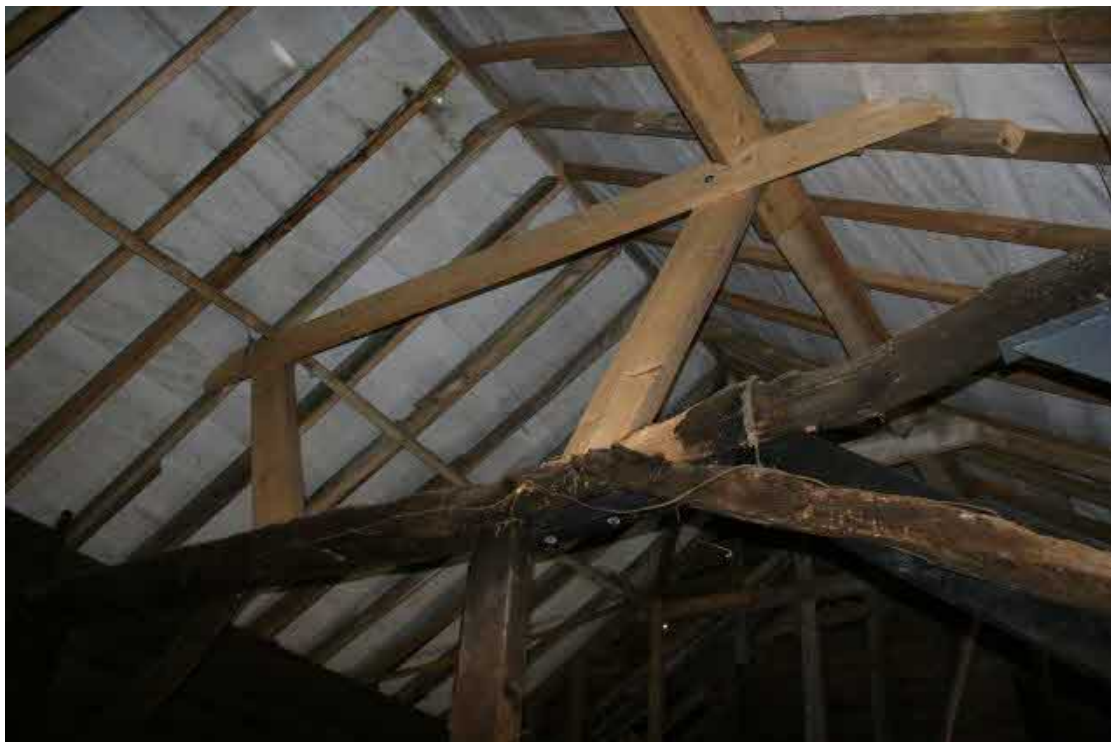
Looking E in the roof of the Workshop.
