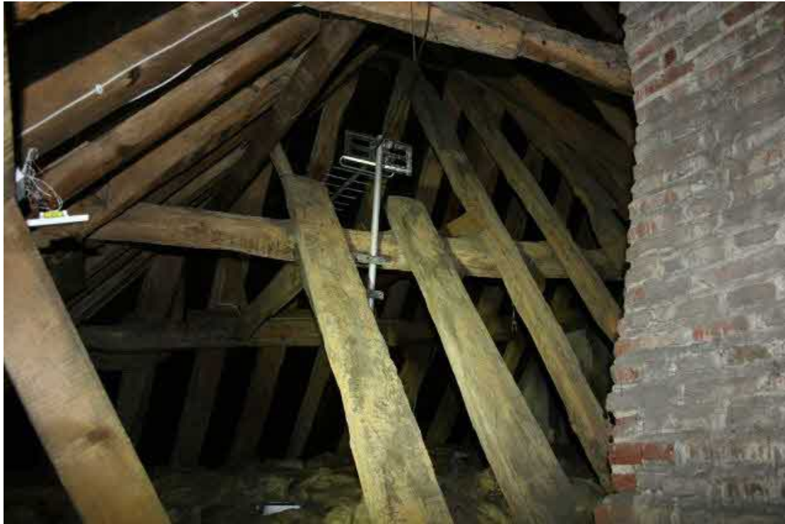
Looking S at the roof over the Cross-wing. West side.
