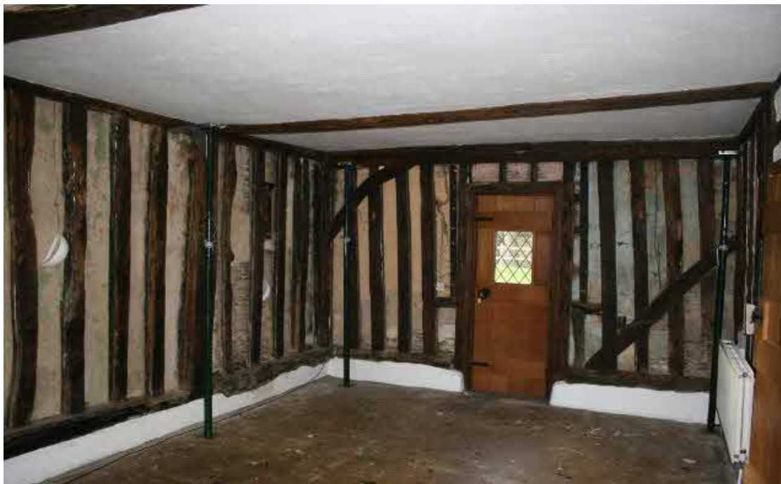
Looking W in the Cross-wing at a former front door.
