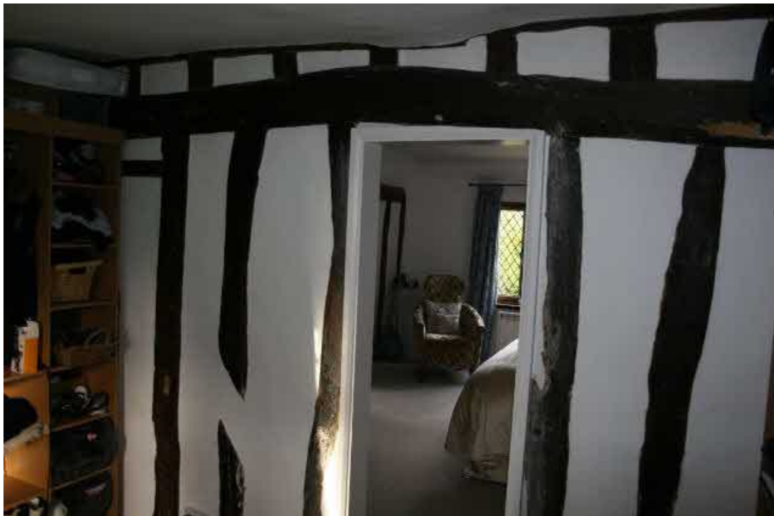
The partition frame in the Cross-wing. Looking E.
