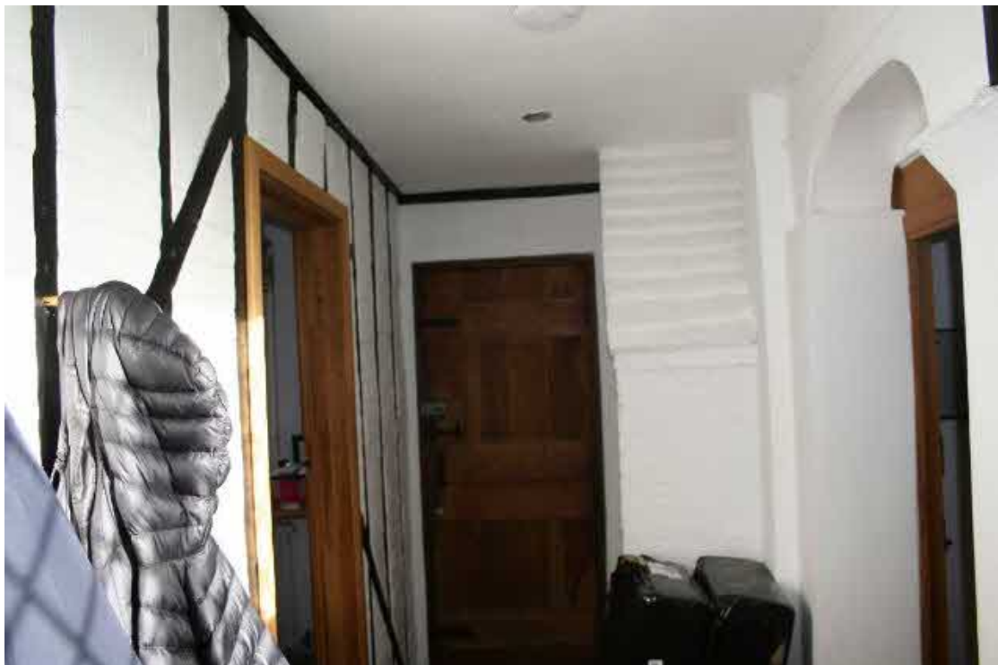
Looking E in the Kitchen hallway. Again note the C19th firestack.
