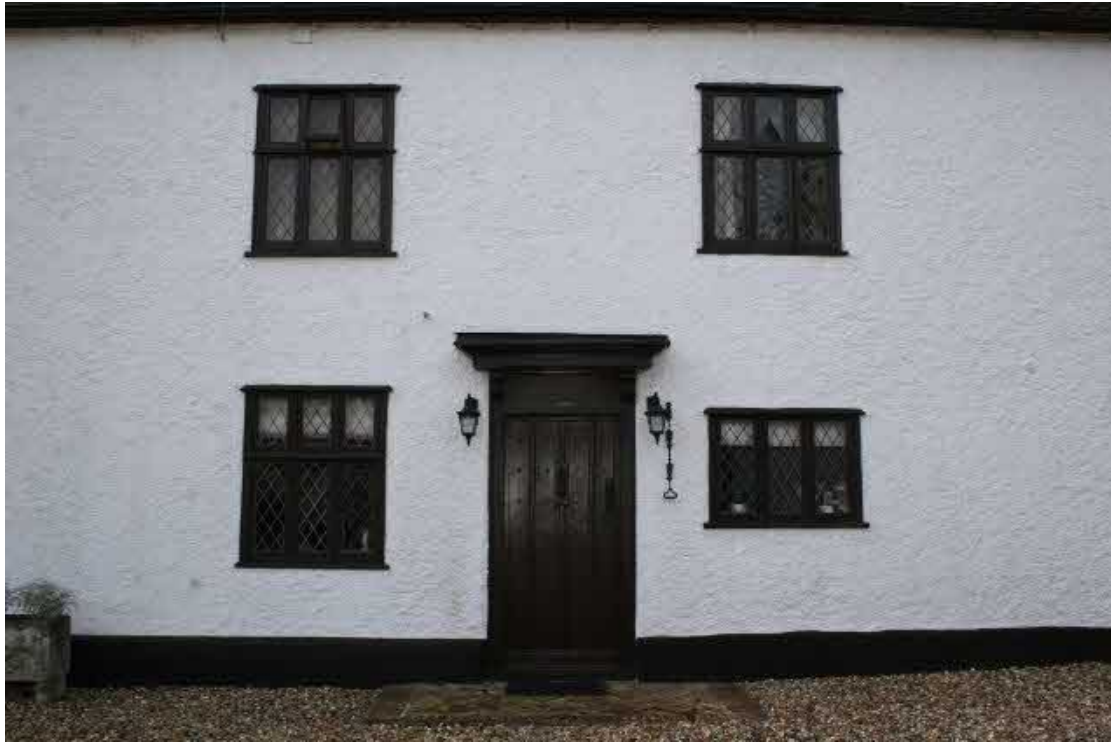
Detail of the front door and windows on the eastern elevation.
