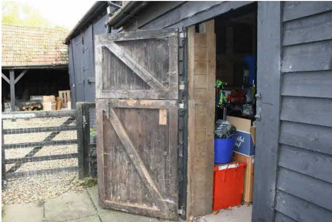
MC20th split stable door rehung in the LC20th with Pozidriv screws.
