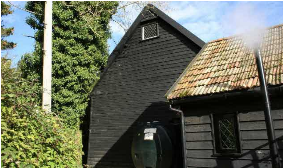
The west elevation of the Listed Barn.
