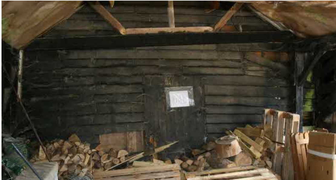
The north elevation of the Workshop retains some original C19th weather-boards.
