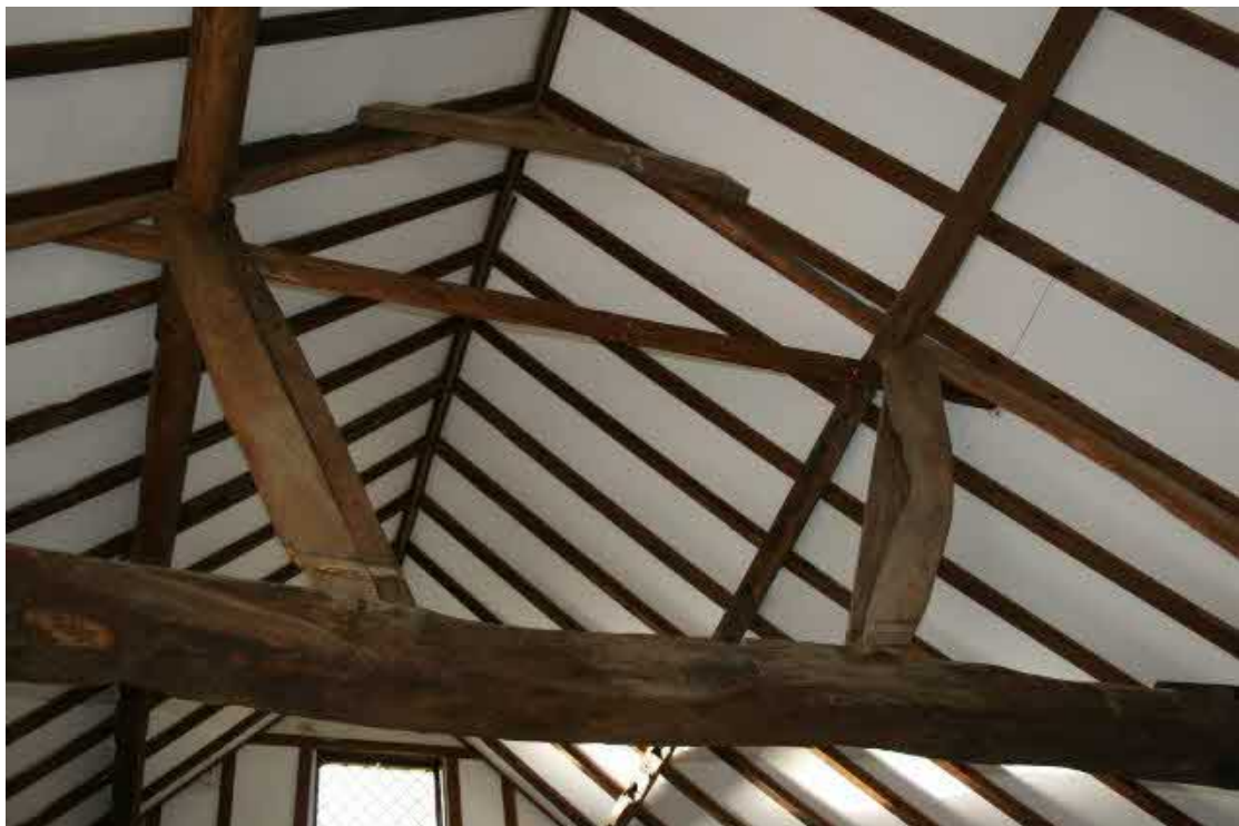
Detail of the westernmost Truss looking NW.
