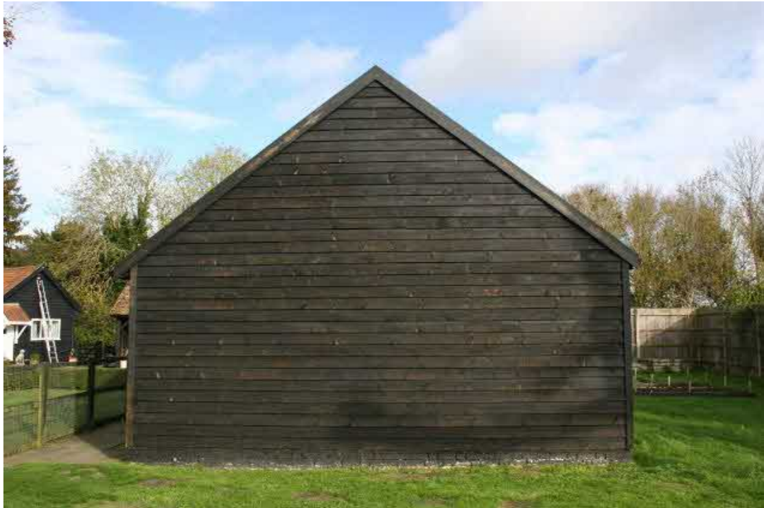
The west elevation of the Stables.
