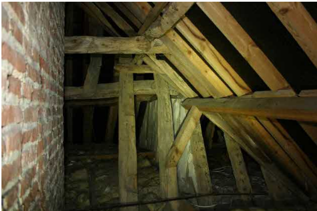
Looking S at the roof over the Cross-wing. East side.
