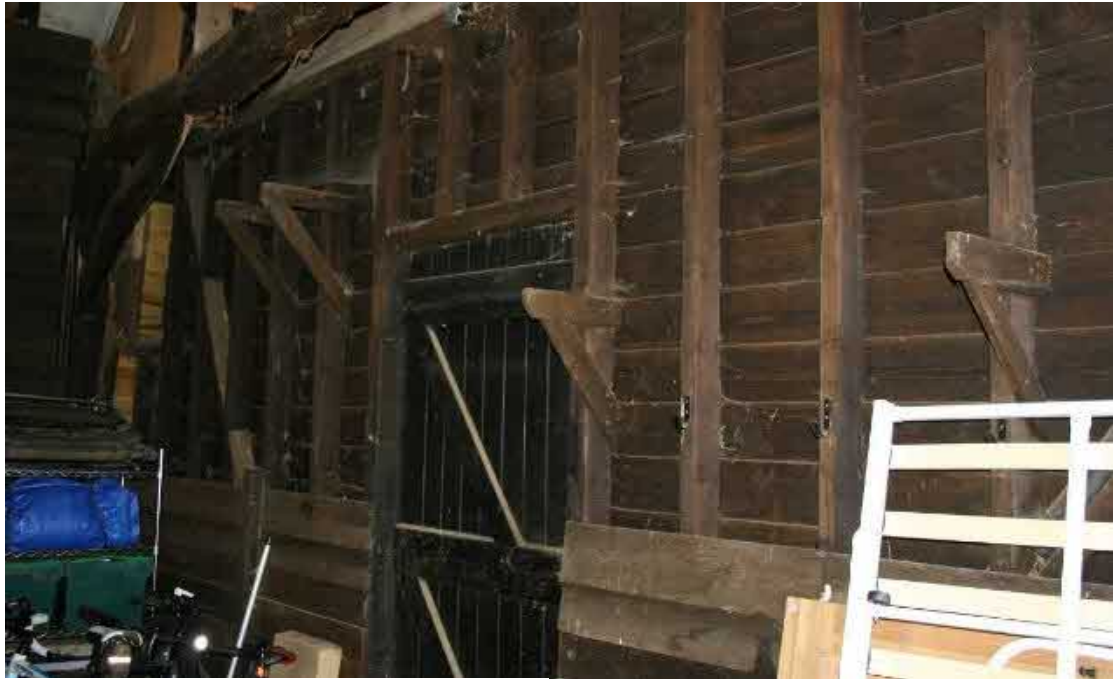
The west wall is built outside of the e-beam.
