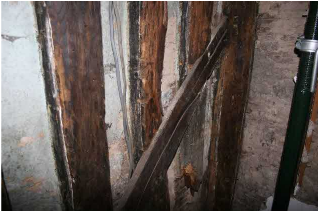
Detail of the brace in the NW corner.
