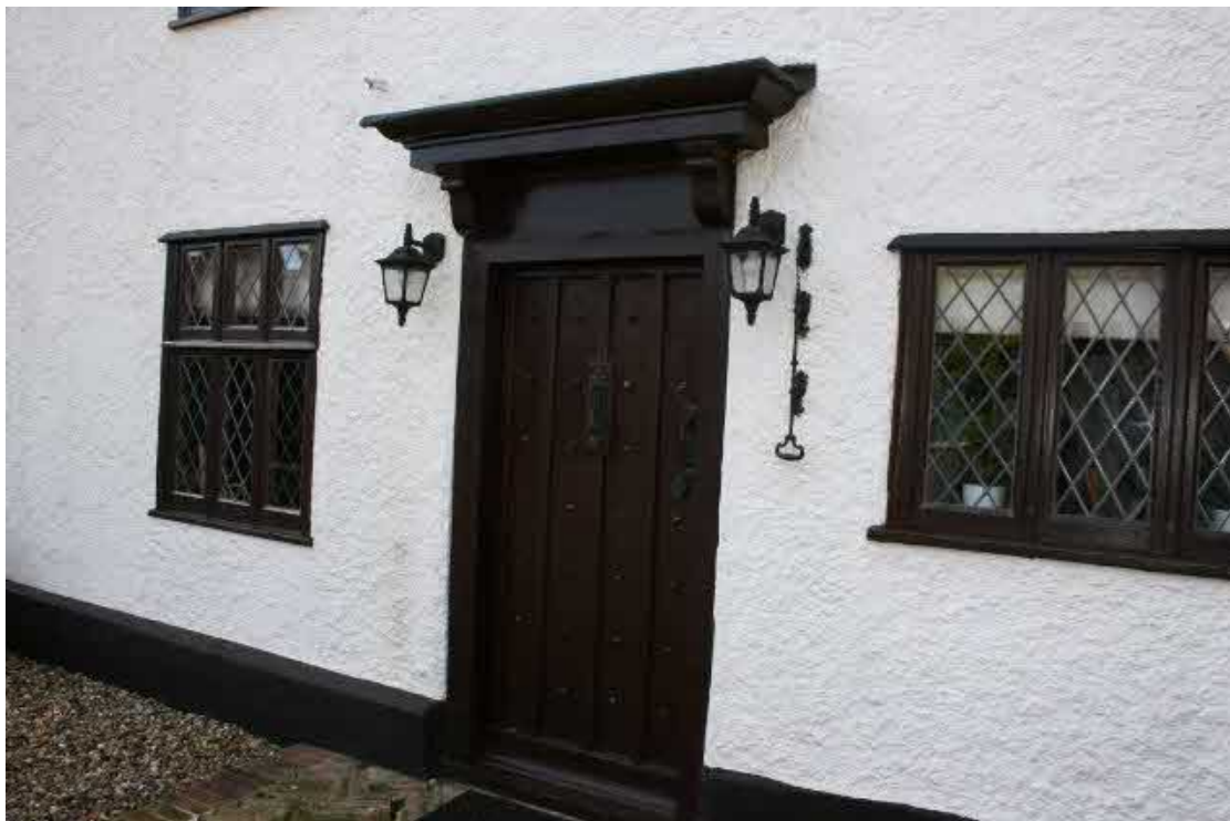
Detail of the front door.
