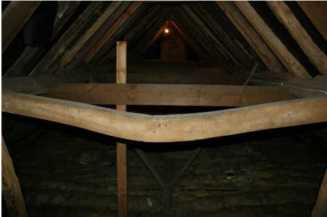
Looking N over the main range at the inverted collar.
