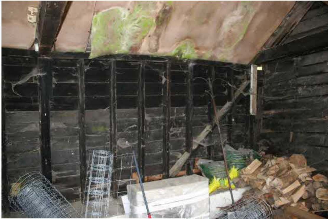
The eastern wall showing the full height 2x4in studs.
