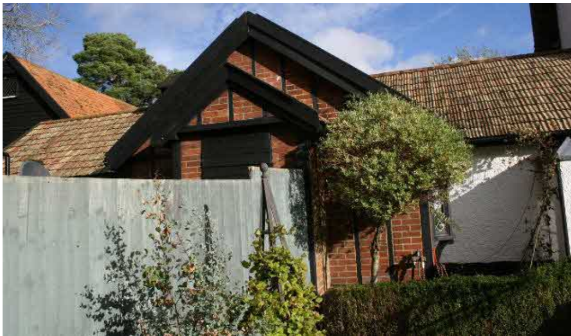
The west elevation with extension to the Kitchen in red brick.
