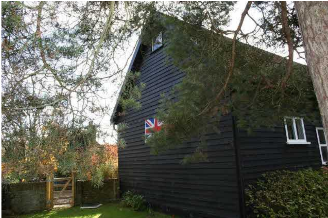
The east elevation of the Listed Barn.
