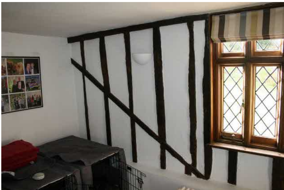
The east wall in the Living Room.
