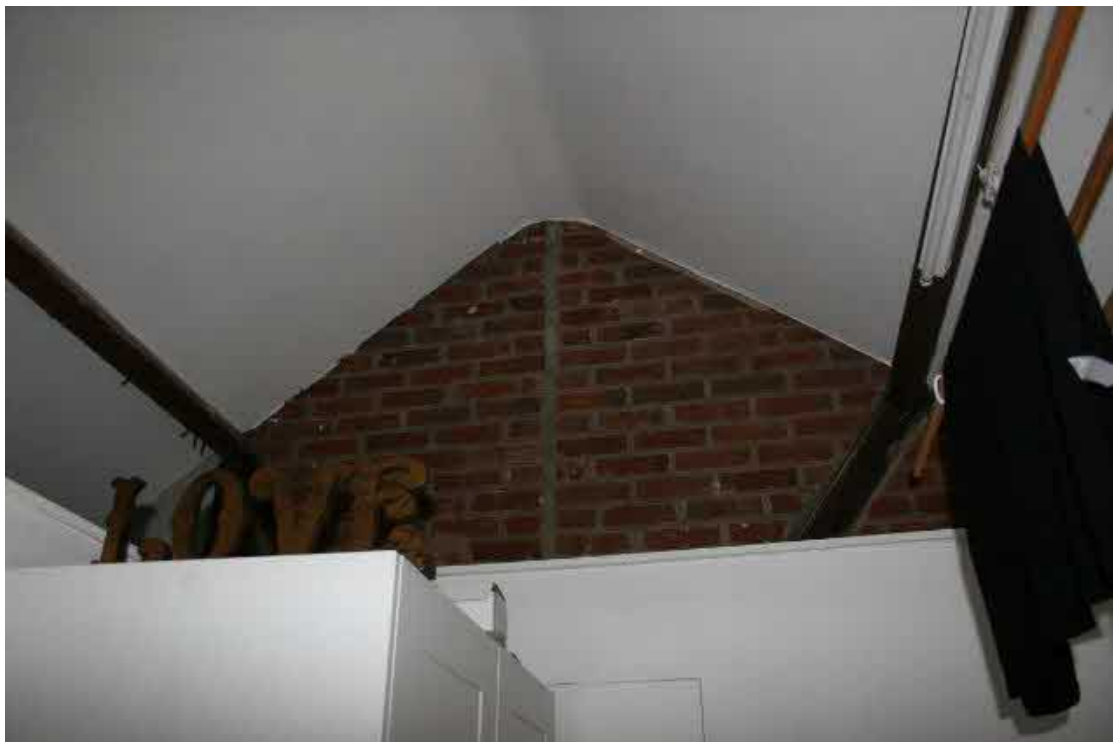
The brick wall seen in the Utility Room is LC20th.
