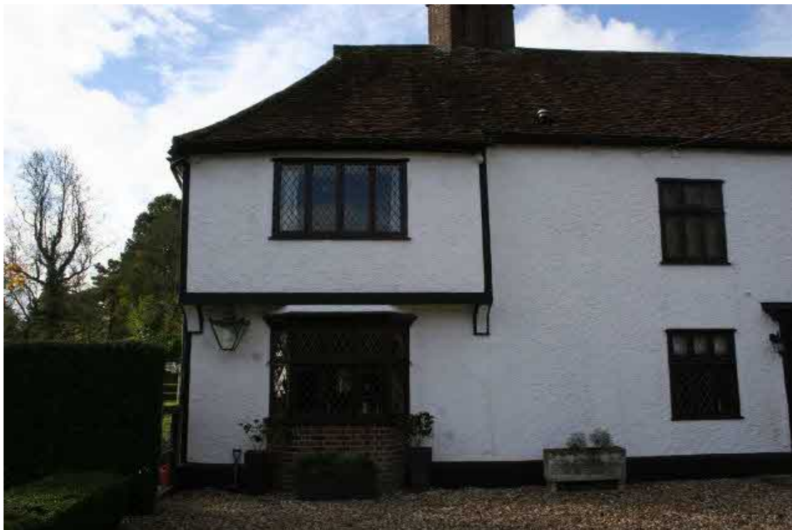
The south cross-wing has an inserted C20th bay window.
