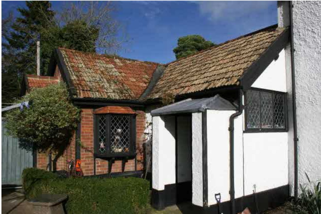
The western extensions to the Kitchen.
