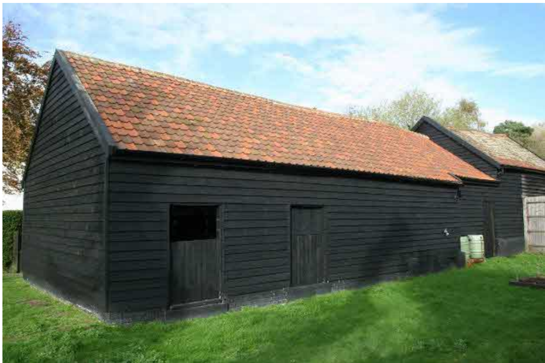
The south elevation of the Stables.
