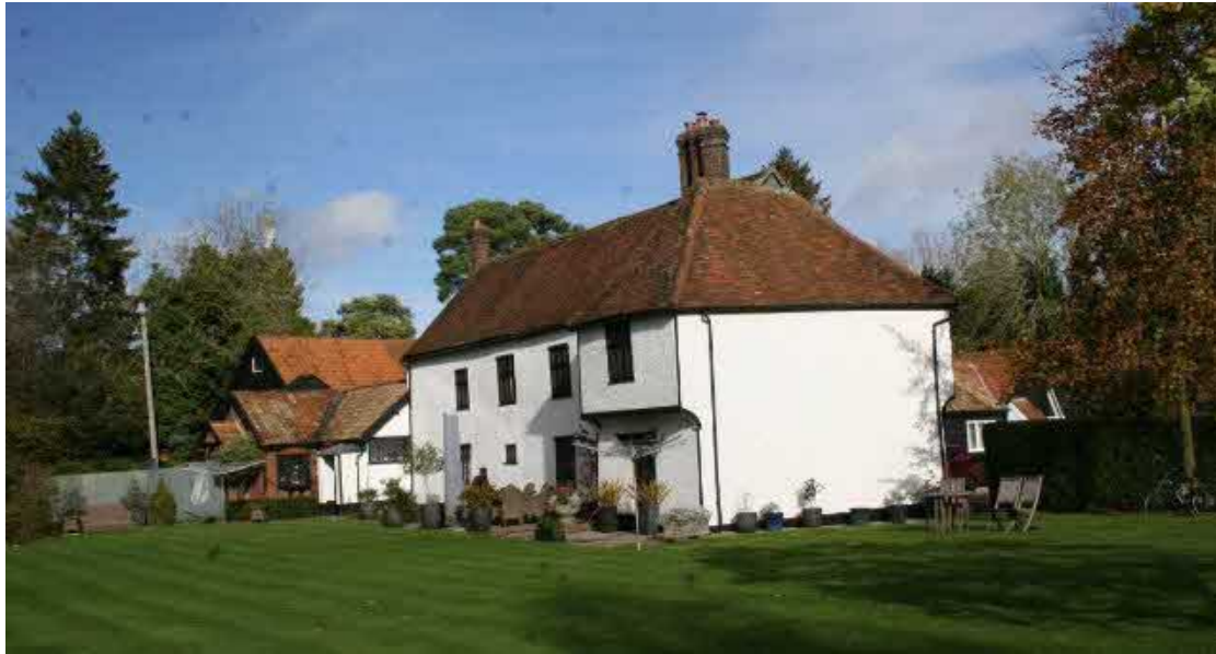
The south and west elevations of the House. The cross-wing is jetted on both sides.
