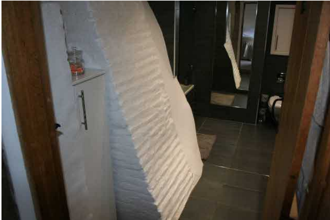
The flank of the firestack seen in the en-suite to Bedroom 1. Looking N.
