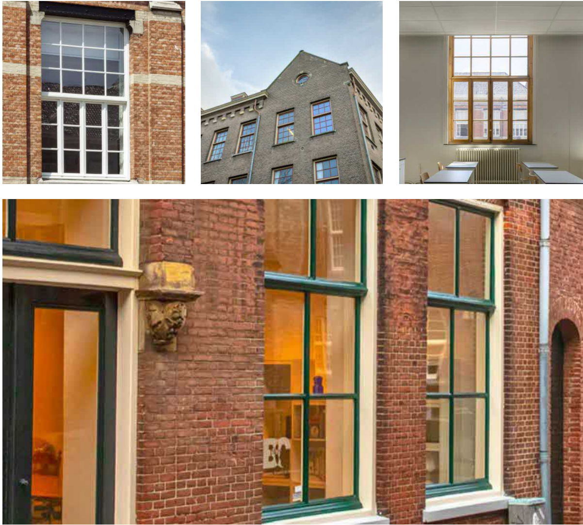
Figs. 19-22 Examples of FINEO vacuum units in traditional buildings (© FINEO)
