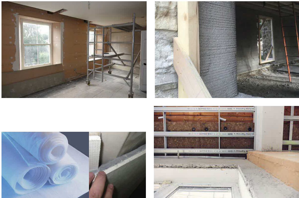
Figs. 29-32 (Clockwise from top left) Woodfibre; insulating lime plaster; combined woodfibre + insulating lime plaster; aerogel (© Nicholas Heath / Bob Prewett / CISL)
