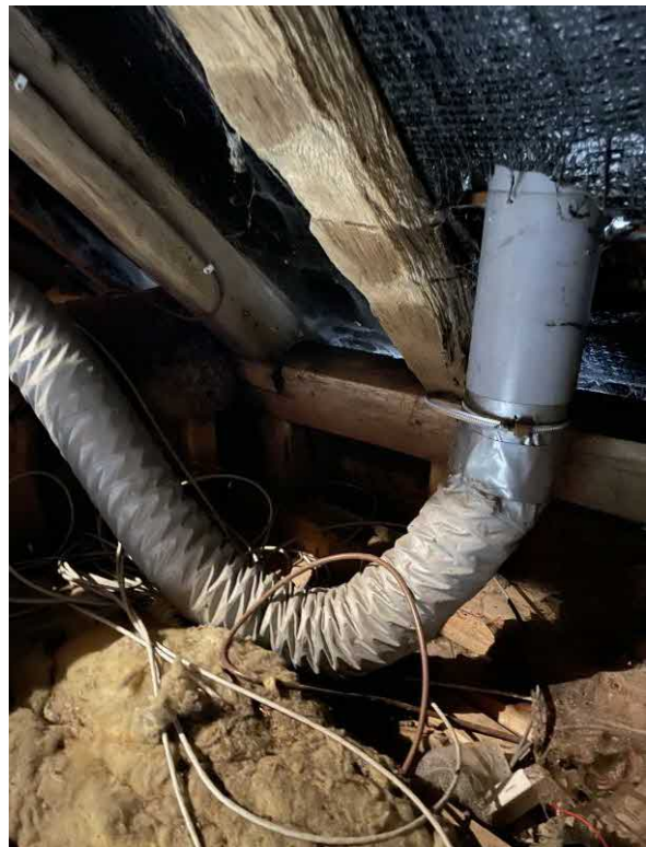
Figs. 33-34 Extract ventilation provision above first-floor wet rooms
