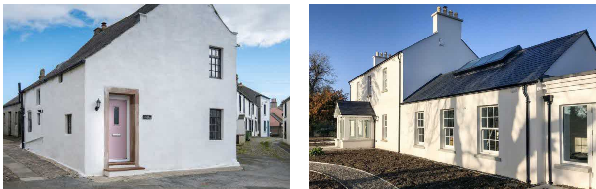
Figs. 27-28 Diathonite systems in Allonby, Cumbria (left) & Clane, Ireland (right) (© Ecological Building Systems)
