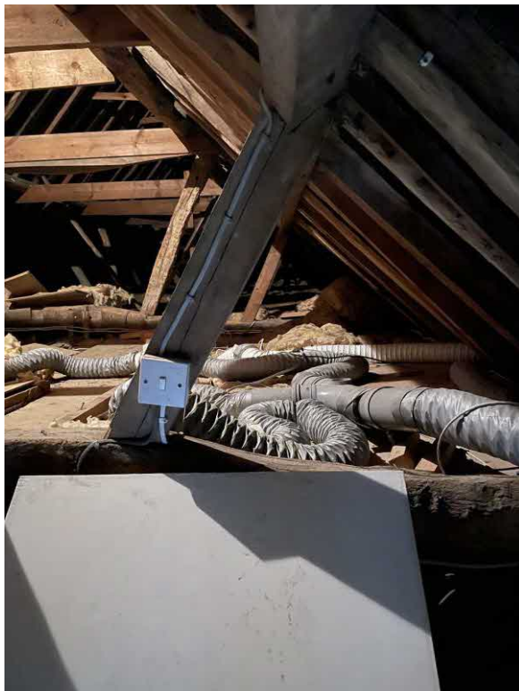
Figs. 33-34 Extract ventilation provision above first-floor wet rooms
