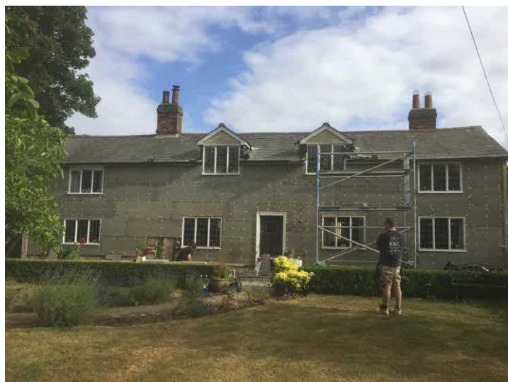
Figs. 25-26 Sheep's wool between timber studs (left); wood wool boards over the top (right) (© Anglia Lime Company)
