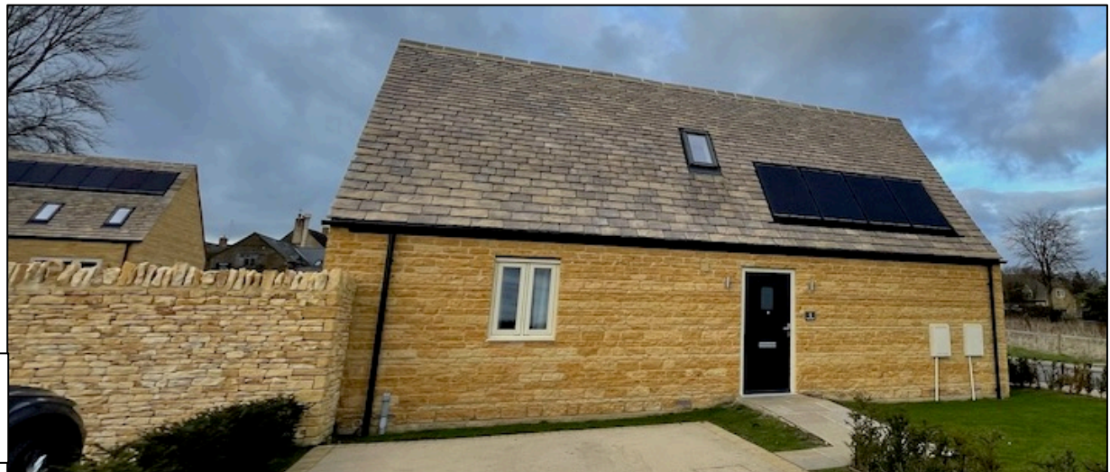
Figure 12: Photographs for context only showing PV panels set flush with the roof coverings.
