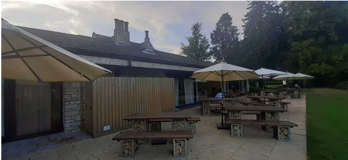
Plate 4: Eastern elevation with its close fitting roof tiles
