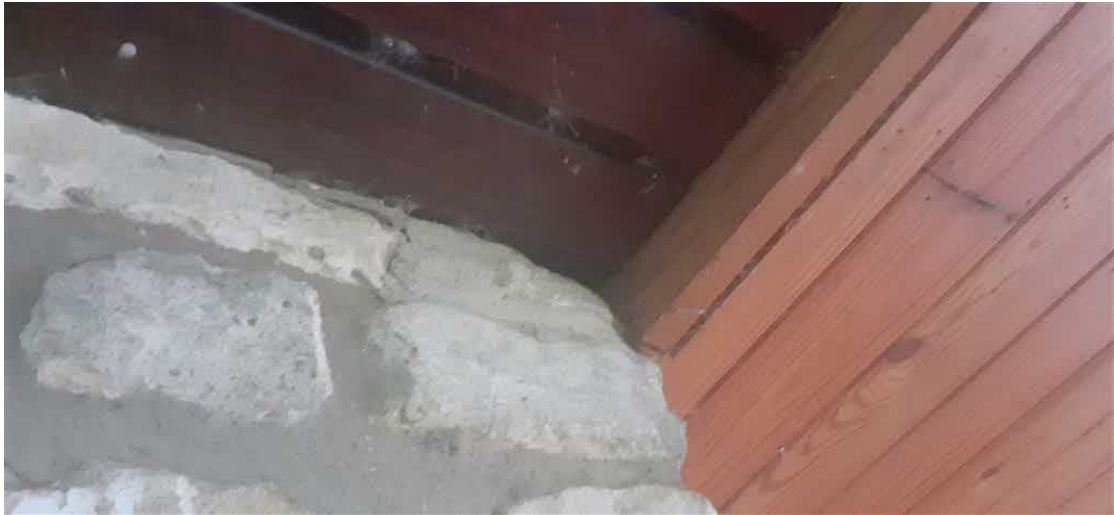
Plates 7: View of a cobwebbed ga on the northern elevation
