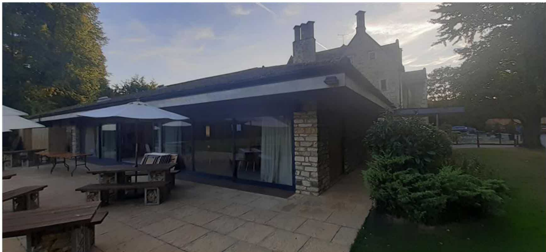
Plate 2: The north-eastern elevation.
