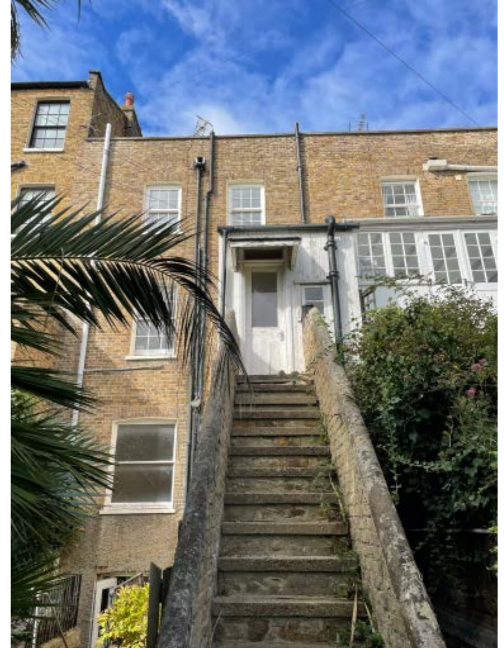
Figure 12. Rear Elevation of House From Garden (Looking North)
