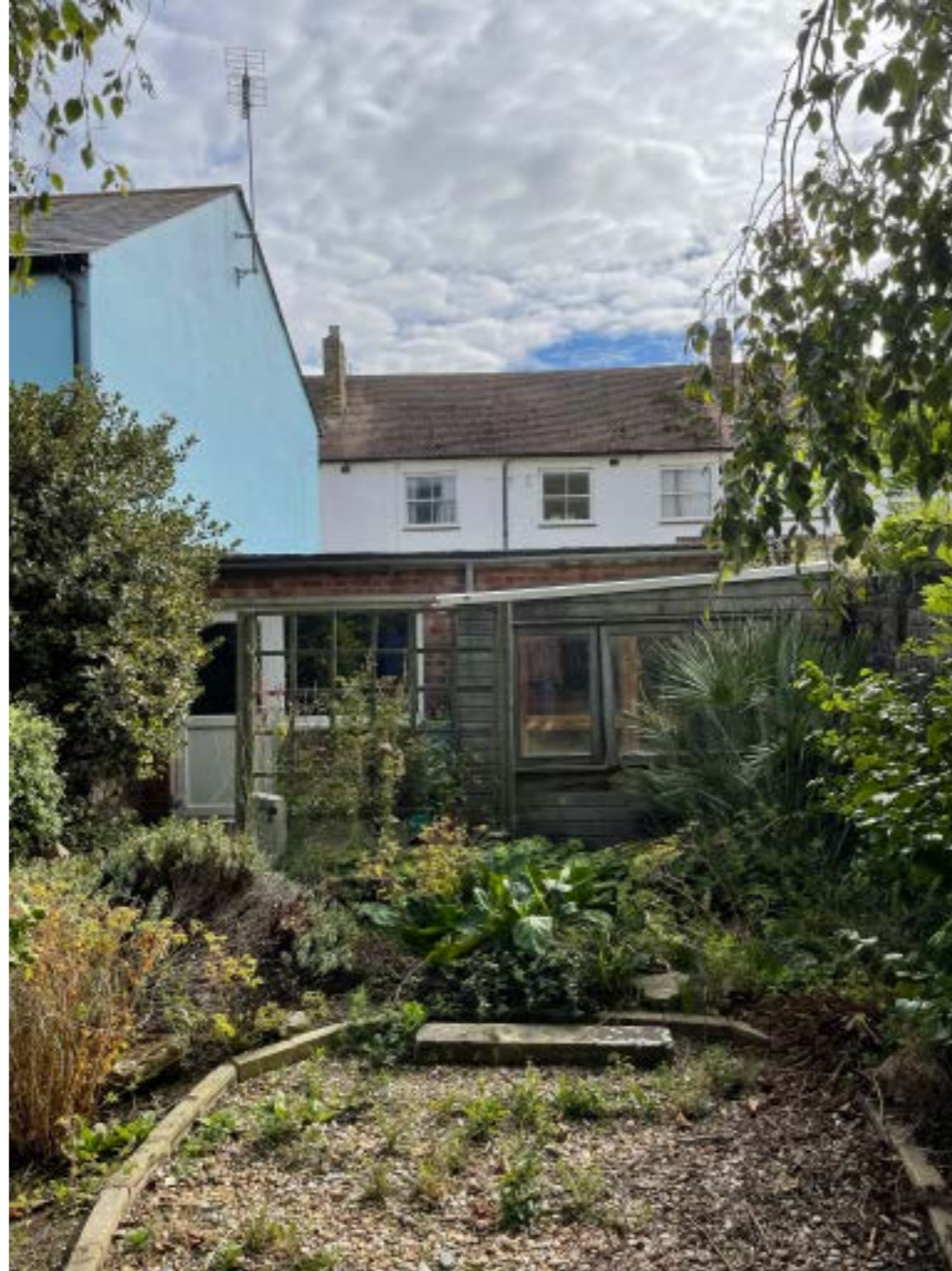
Figure 11. Rear Elevation of Garage From Garden (Looking South)
