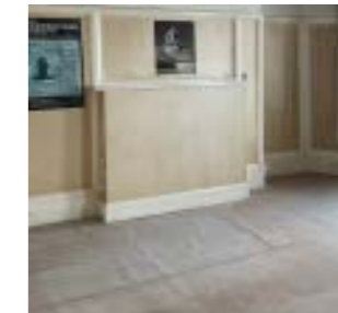
Second Floor Front
