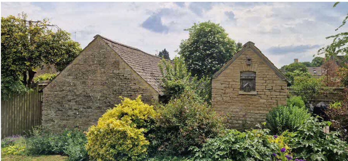
outbuildings - garden elevation (north)
