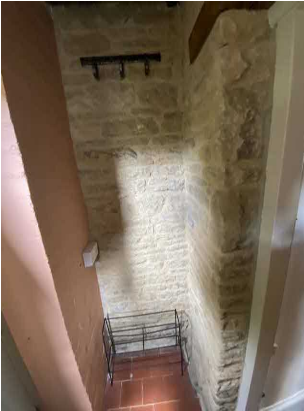
rear porch, erected 1996 (proposed wc)
