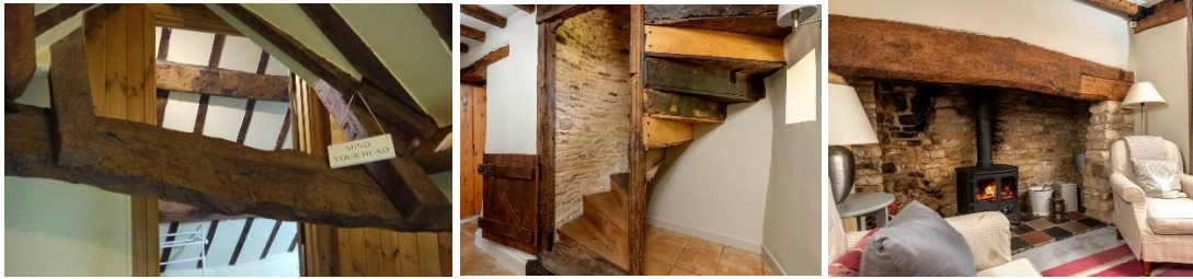
Plate 6 (left) Historic timber beams to second floor, plate 7 (centre) historic spiral staircase and plate 8 (right) fireplace to main living room.
