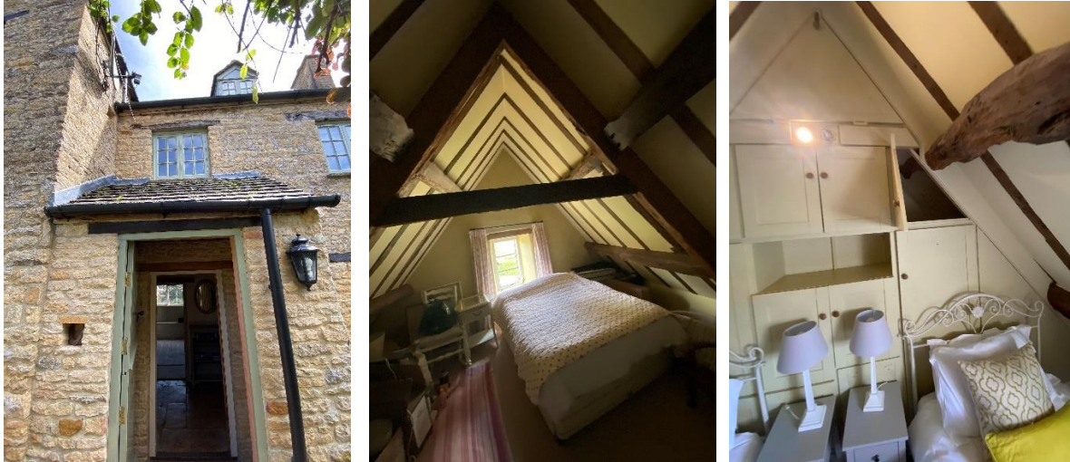
Plate 12 (left) Modern porch proposed to be converted to WC, plate 13 (Centre) Bedroom and proposed rooflight and plate 14 (right) cupboards proposed for removal to create en-suite.
