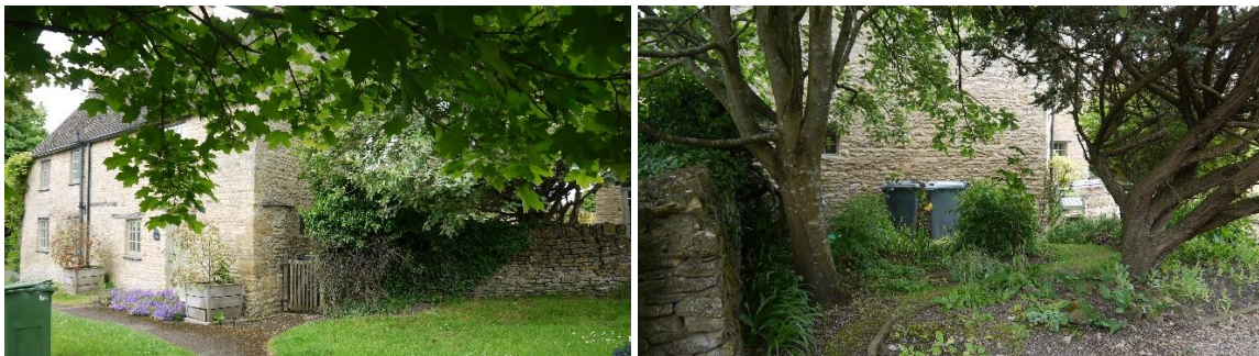
Plate 10 (left) view of property from Hackers Lane and existing stone boundary wall. Plate 11 (right) proposed location of extension onto side gable and area of stonework to be removed for access.
