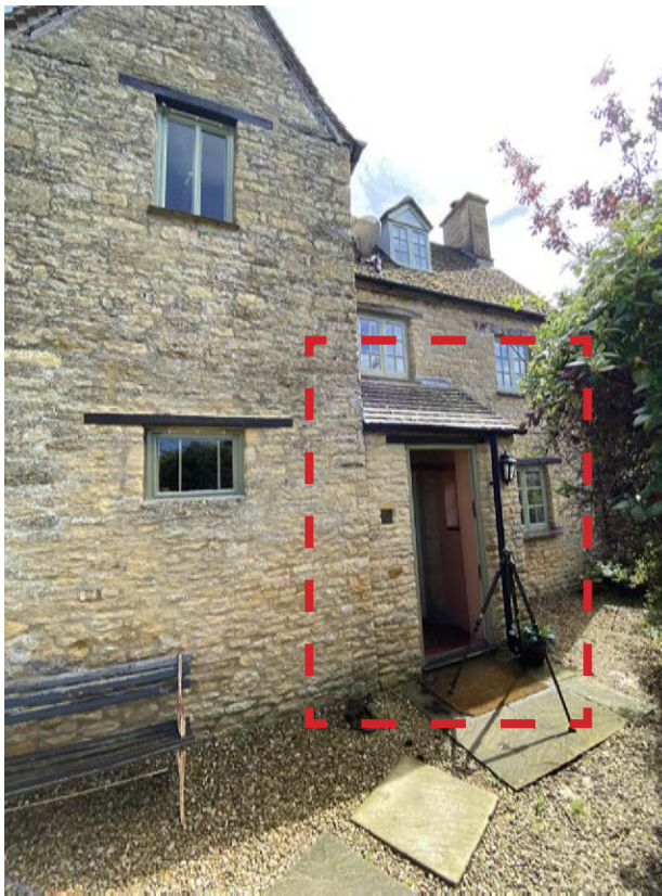
rear porch, erected 1996 (proposed wc, doorway to be infilled with timber cladding)
