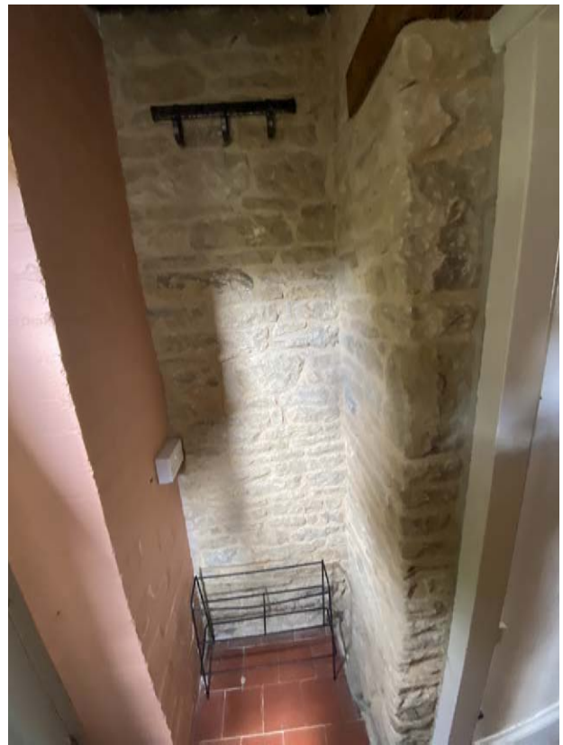
rear porch, erected 1996 (proposed wc)
