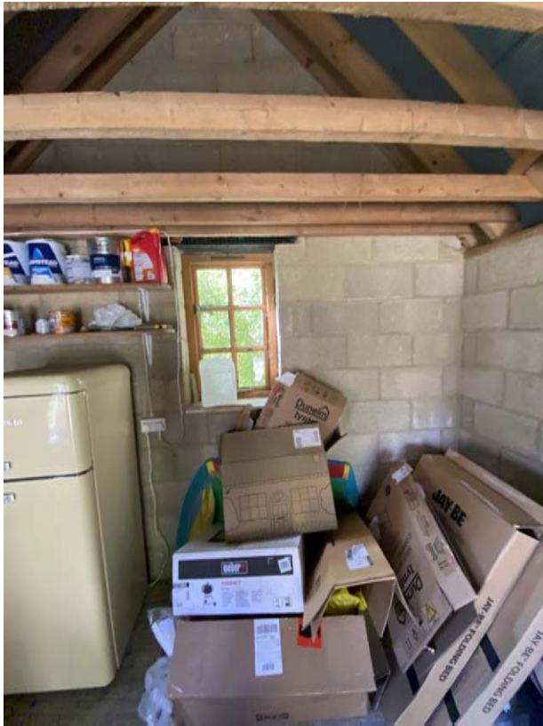
garage - rear gable interior - proposed bat loft to be formed over
