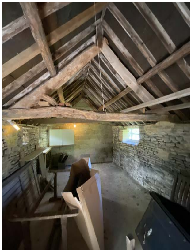
outbuilding - existing stonework repaired and repointed, blockwork party wall dry-lined in new shower room at end - modern concrete slab floor rained or replaced tbc
