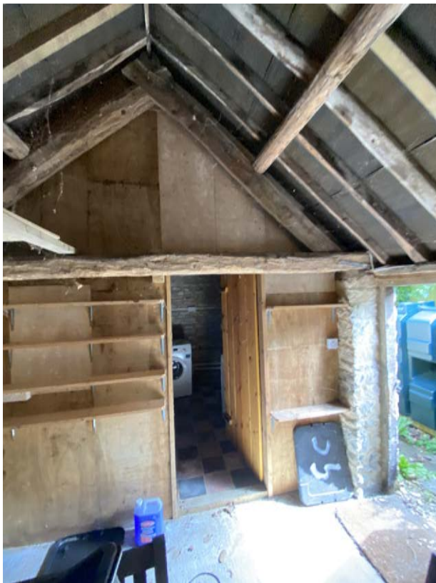
outbuilding, renovated and reroofed 2001, partition and shelves to be removed
