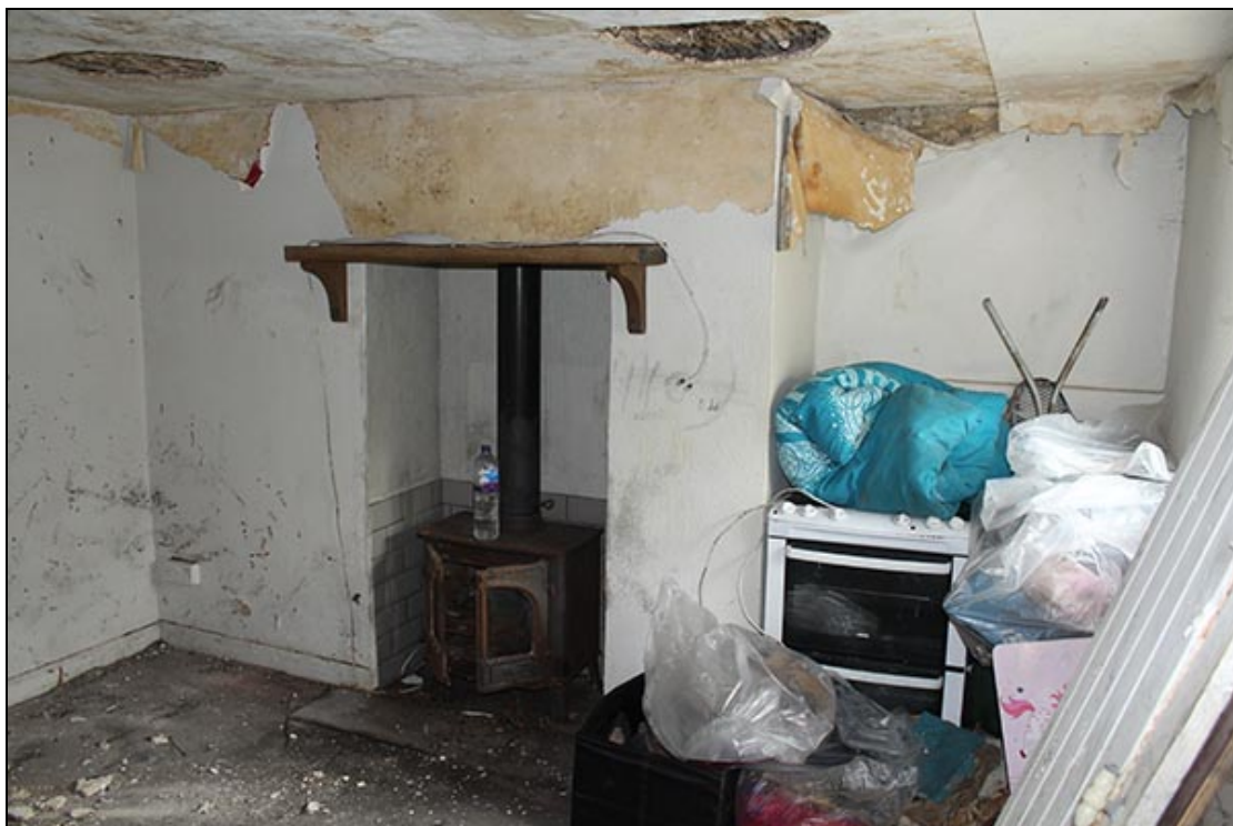
Figure 15 Ground floor fireplace in the front room of No.1, looking east
