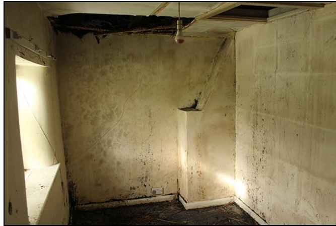
Figure 16 The first floor fireplaces now lie blocked up just to the left of the right hand Phase 4 wall, here seen in No.2, looking west
