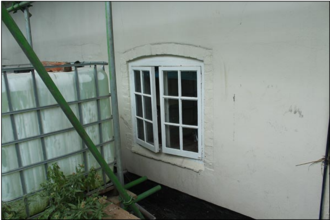
Figure 27 A typical Phase 3 window, with bevelled sill
