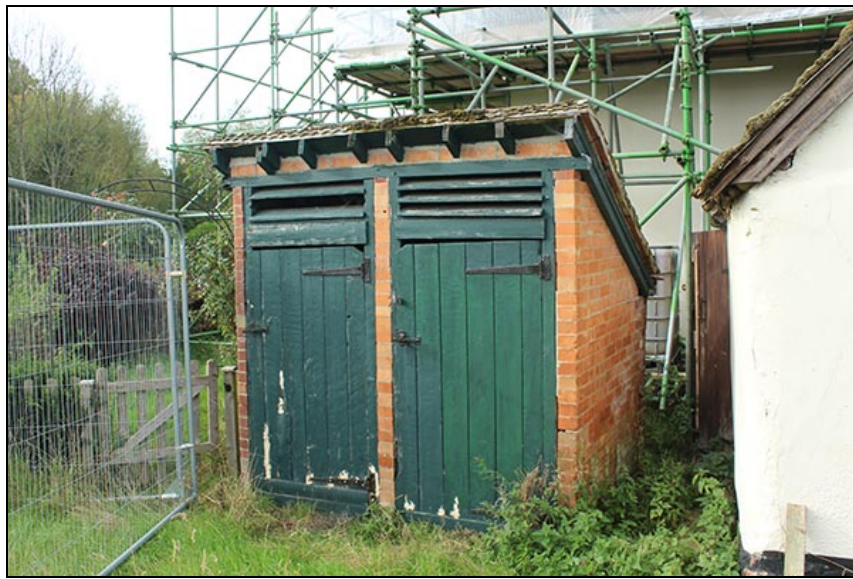
Figure 24 The eastern pair of new brick privies of Phase 3, looking west
