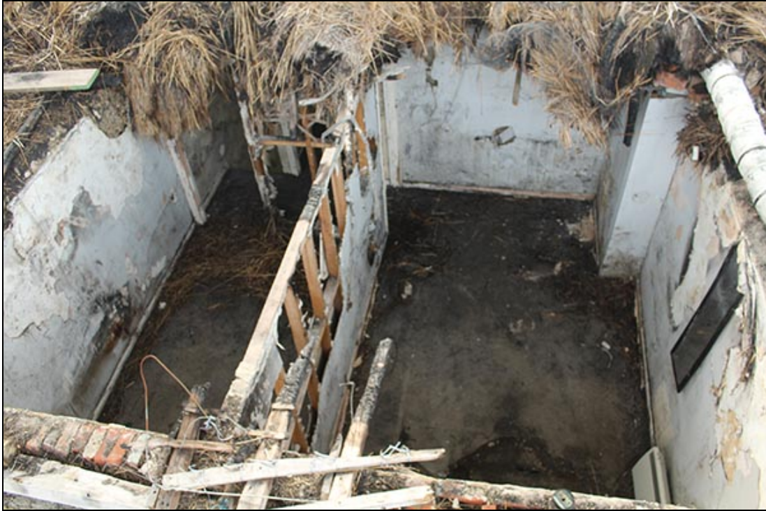
Figure 33 The new first floor layout of Phase 4, here in No.2, looking south
