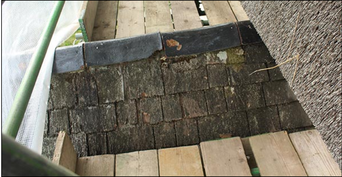
Figure 29 The Phase 3 ridge tiles over the eastern outshot, looking south
