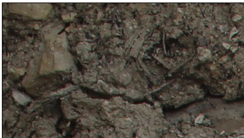
Figure 13 Detail of the chalk cob walling
