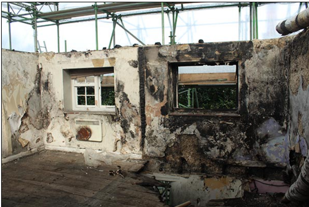
Figure 32 New Phase 4 windows, with quarry tiles laid in the sills, in the first floor rear wall of No.1, looking north
