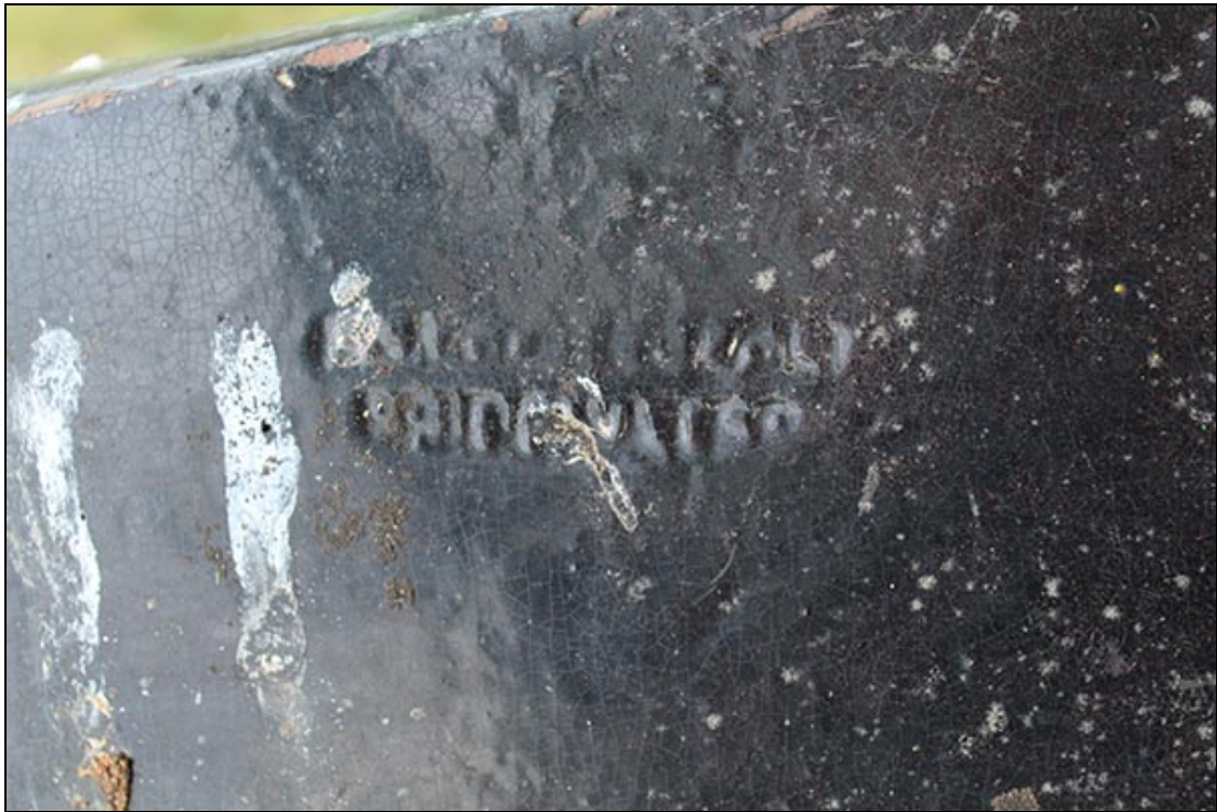
Figure 30 Detail of one of the Phase 3 ridge tiles, showing the maker's stamp
