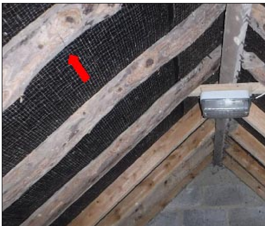
Figure 22 Tarred twine mark on one of the rafters of the eastern outshot, indicating that it was once thatched like the neighbouring cottages, looking east
