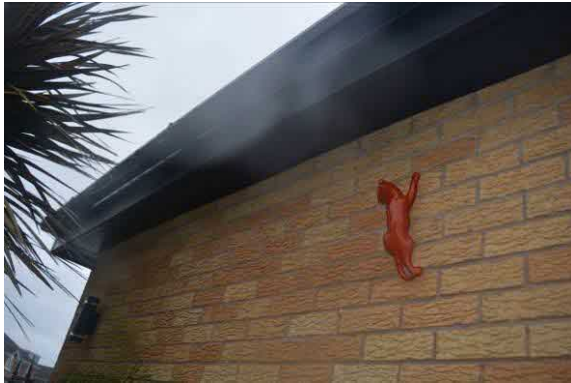
Figs. 5 & 6 UPVC soffits fully sealed with no gaps/crevices present
