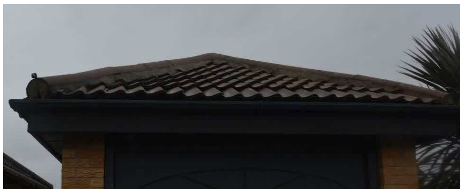
Fig. 4 External roof detail – no gaps/crevices present
