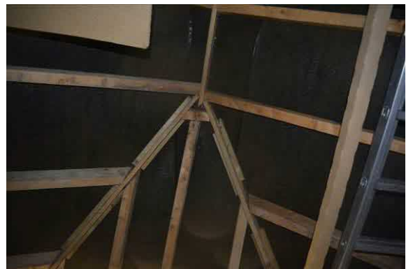
Figs. 7 & 8 Roof structure with felt lining
