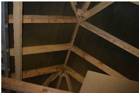
Figs. 7 & 8 Roof structure with felt lining
