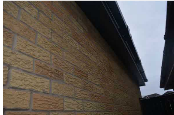
Figs. 5 & 6 UPVC soffits fully sealed with no gaps/crevices present
