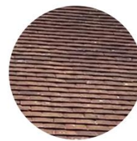
Clay Tile Rood Finish (Existing)
