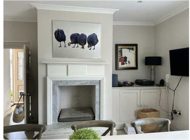
Photo of wall and cupboard to be removed
