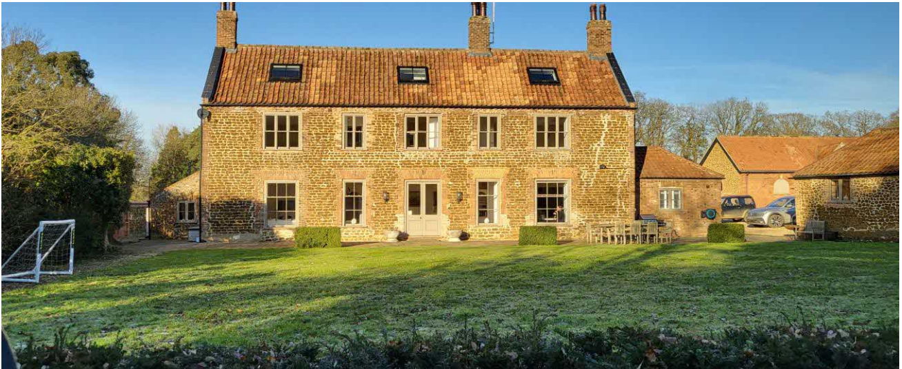
Photo of South elevation following renovation under 15/00095/LB (taken in 2023)
