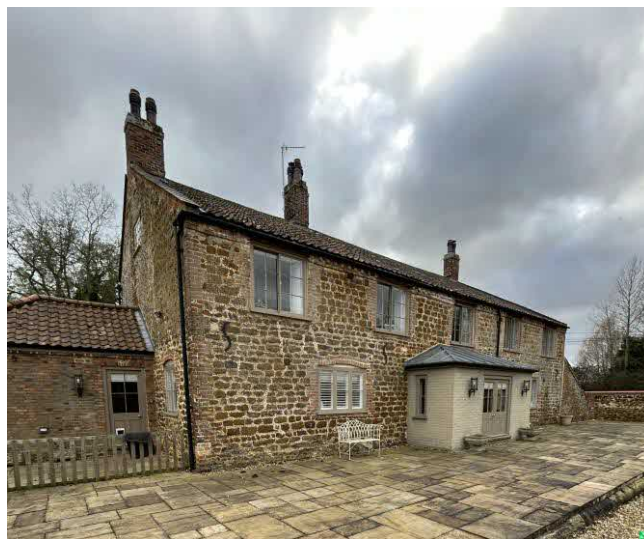
Photo of North elevation following renovation under 15/00095/LB (taken in 2023)
