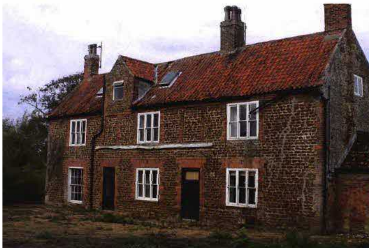
Photo of South elevation prior to renovation in 2010
