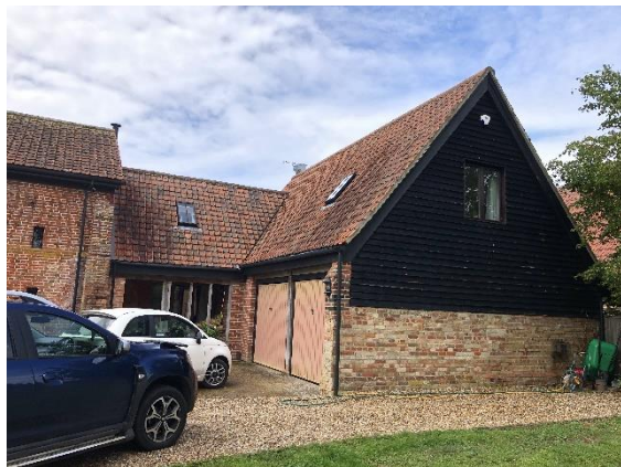
House looking west. Proposed area for lean-to garage
