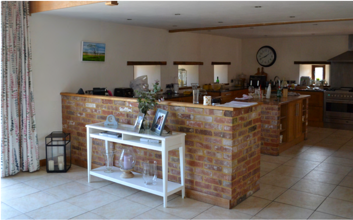
Plate 10 - Kitchen dwarf wall to be removed.
