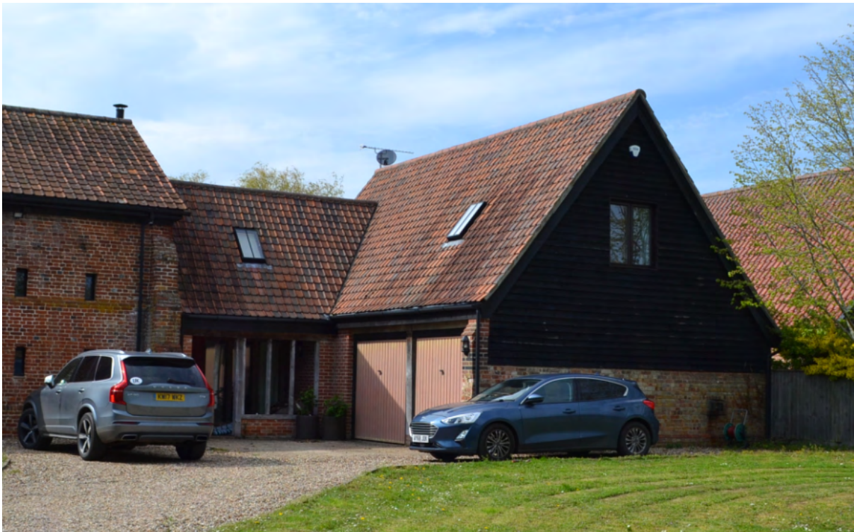
Plate 8 - The front porch and attached garage at present.
