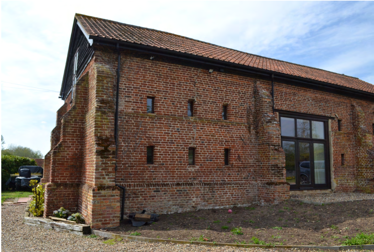
Plate 5 - Buttressing, Plinth and Offset & Ventilation Loops
