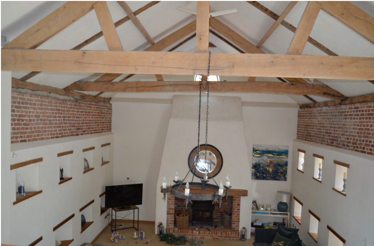
Plate 6 - Existing and replacement roof structure, chamfered ventilation loops
