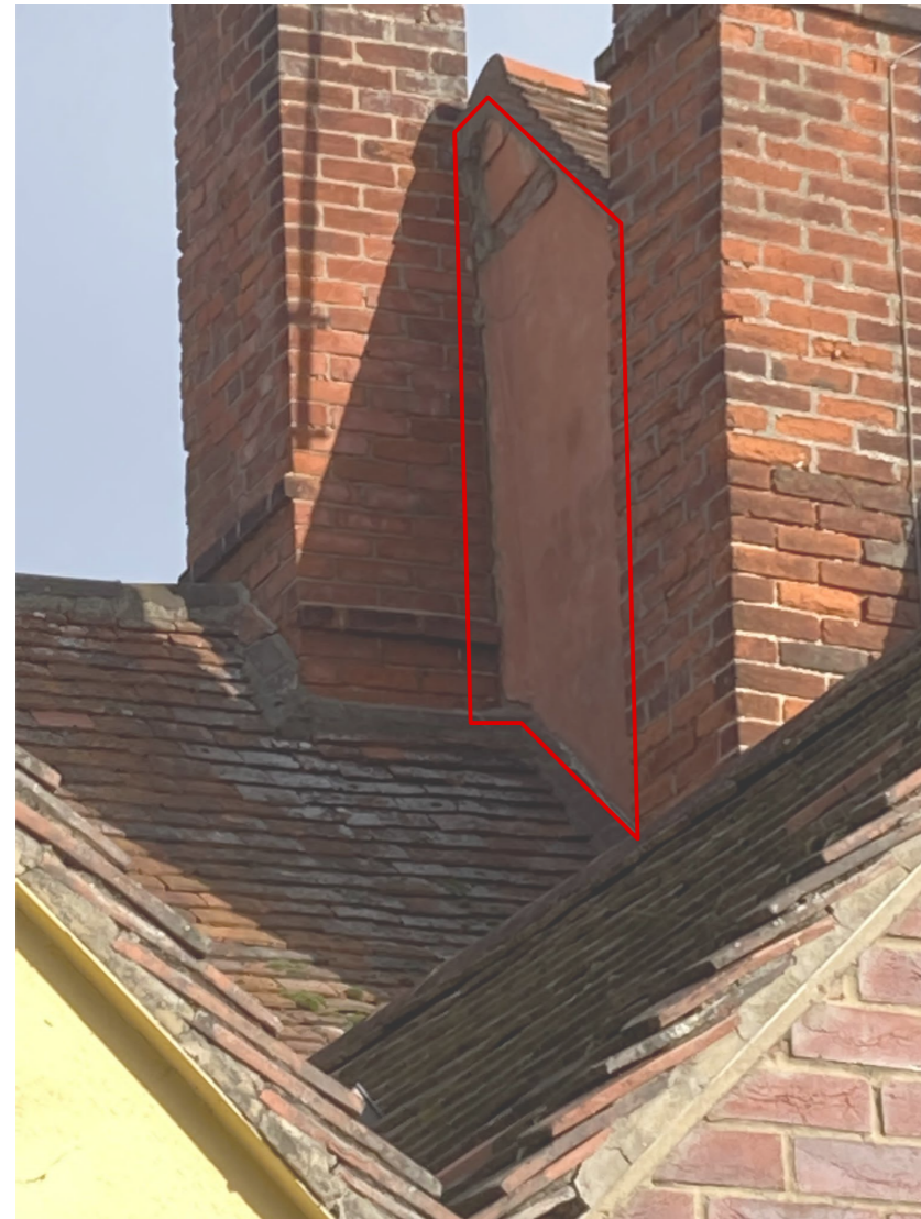
Remove and replace the lath and lime render between the two chimneys with an orange lime render to match.
