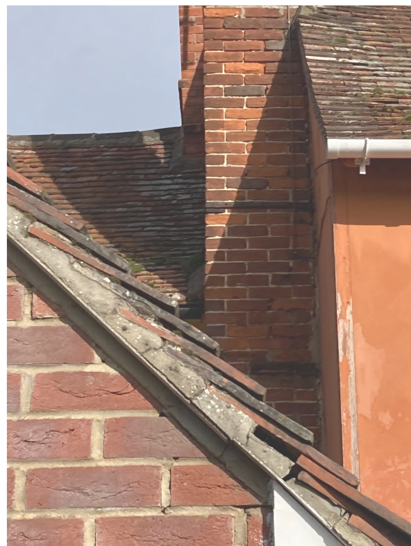
Remove and replace the lath and lime render between the two chimneys with an orange lime render to match.
