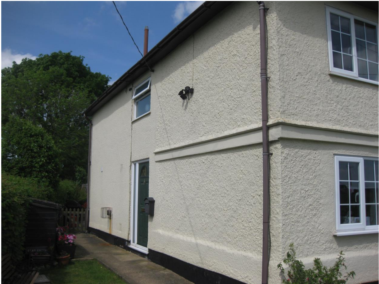
Photograph 1: Location for Proposed Installation of a New Porch at 36 Cooper Road.
