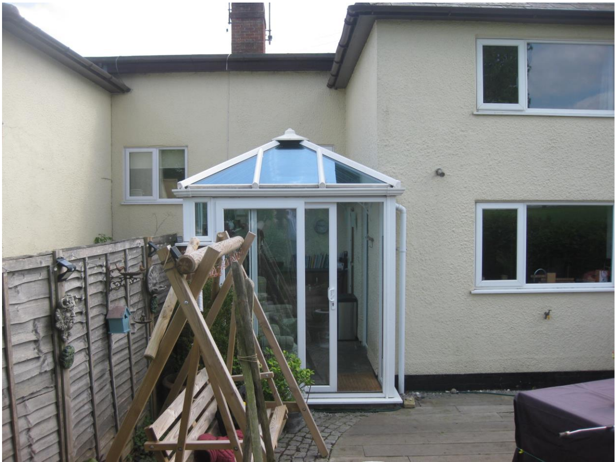
Photograph 2: Location for proposed extension to replace the conservatory at 36 Cooper Road.
