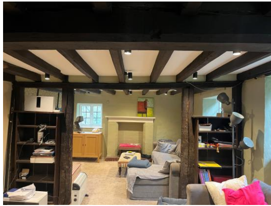
Figures 8 and 9: Photographs showing the exposed timber framing at ground and first floor level
