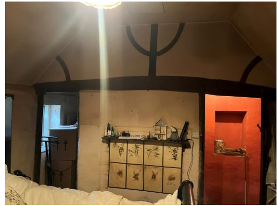
Figures 8 and 9: Photographs showing the exposed timber framing at ground and first floor level
