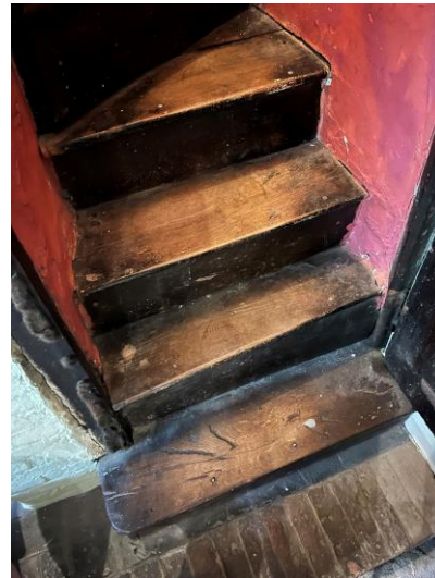
Figures 10 and 11: Historic winder staircase located within the historic core of the building
