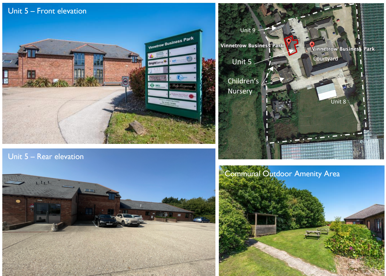
Figure 1 – Aerial photograph and images of the site / wider context
