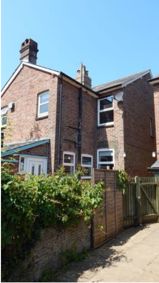
Image 04 - Rear Elevation of No4, No5 to the right.
