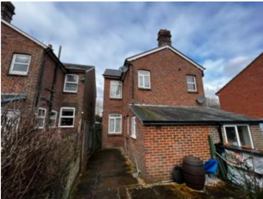
Image 03 - Rear Elevation of No5, No4 to the left, No6 to the right
