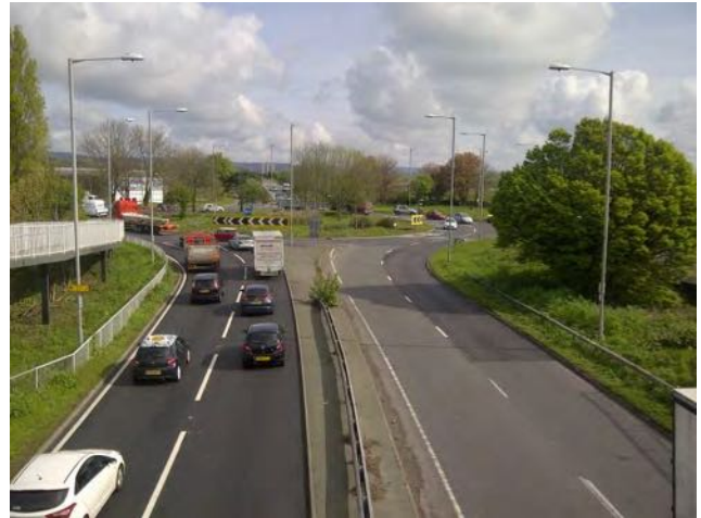
A27 south-west of the A259 Bognor Road Roundabout
