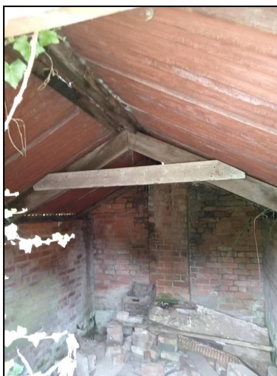
Photo 6 – Internal view of B4
