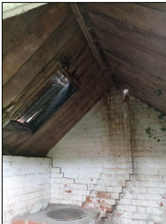
Photo 5 – Internal view of B3
