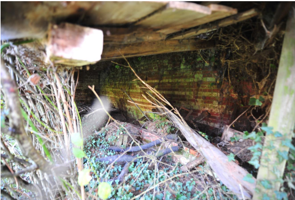
Pl.6: The interior of the former glasshouse
