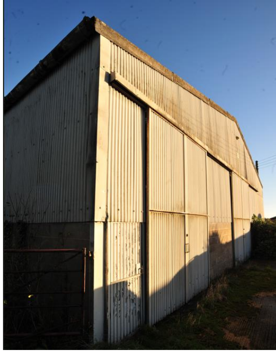
Pl.7: The east elevation of the modern Barn viewed from the lane.
