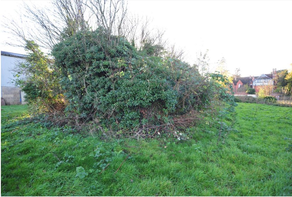
Pl.5: The overgrown derelict glasshouse from the east, Meredith in the background.
