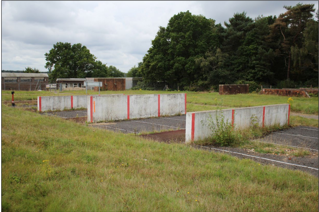
Photo 64: Apparatus Feature B10, viewed from the north-east
