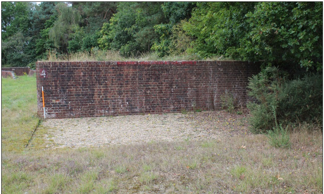
Photo 25: Apparatus Feature A6, viewed from the north-east.
