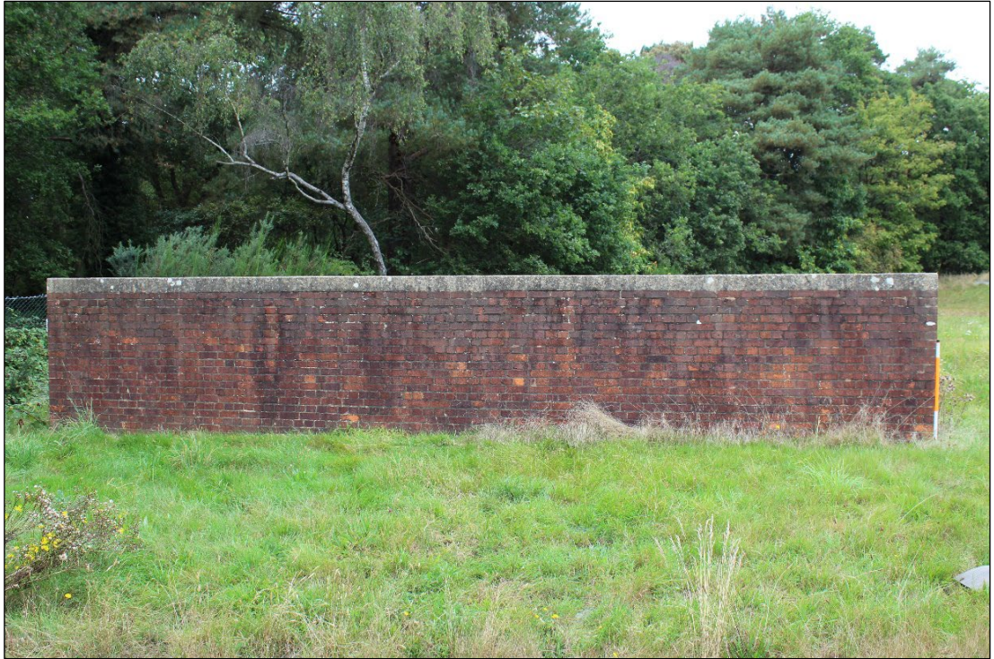
Photo 14: Apparatus Feature A3, viewed from the south
