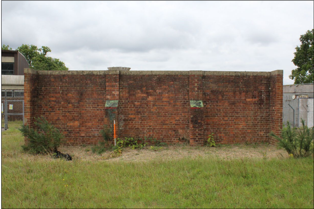
Photo 11: Apparatus Feature A1, viewed from the north
