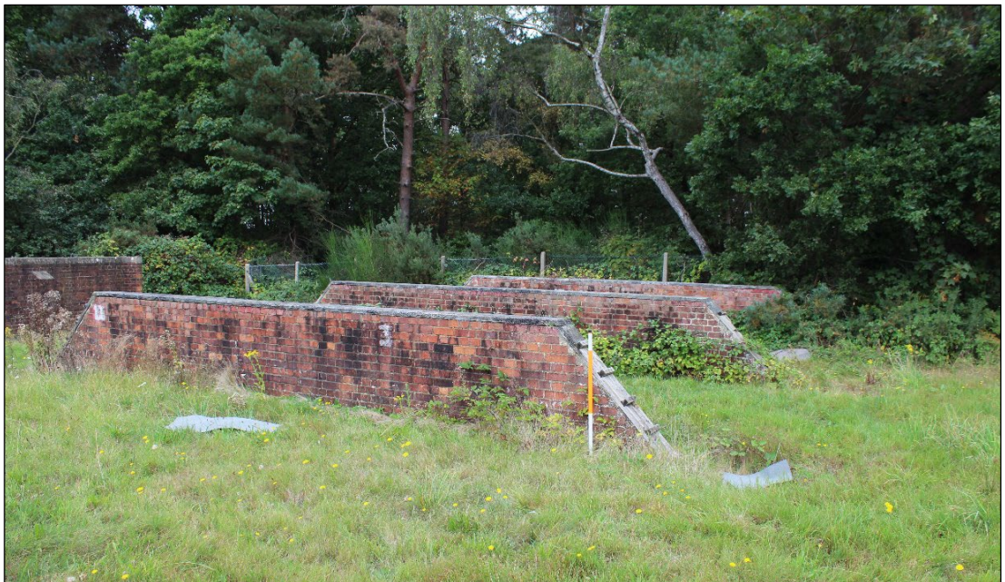
Photo 18: Apparatus Feature A4, viewed from the north-east
