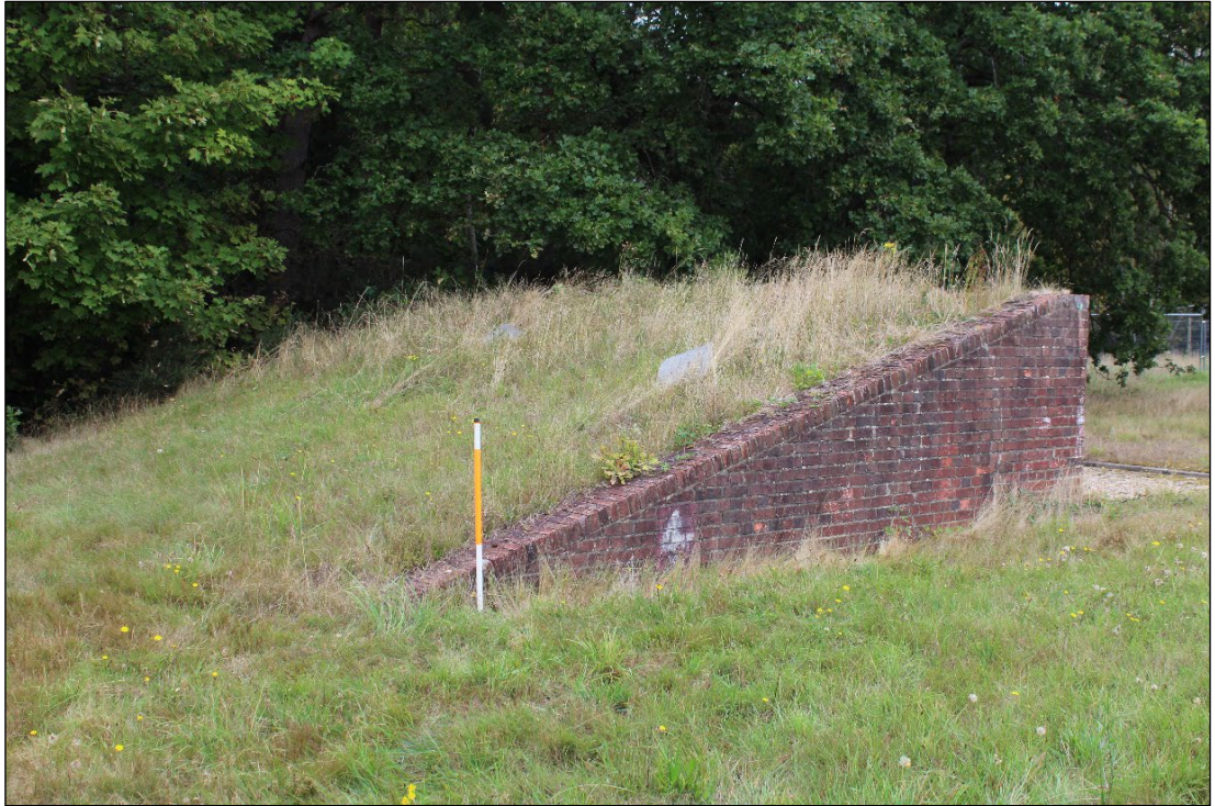
Photo 22: Apparatus Feature A6, viewed from the south
