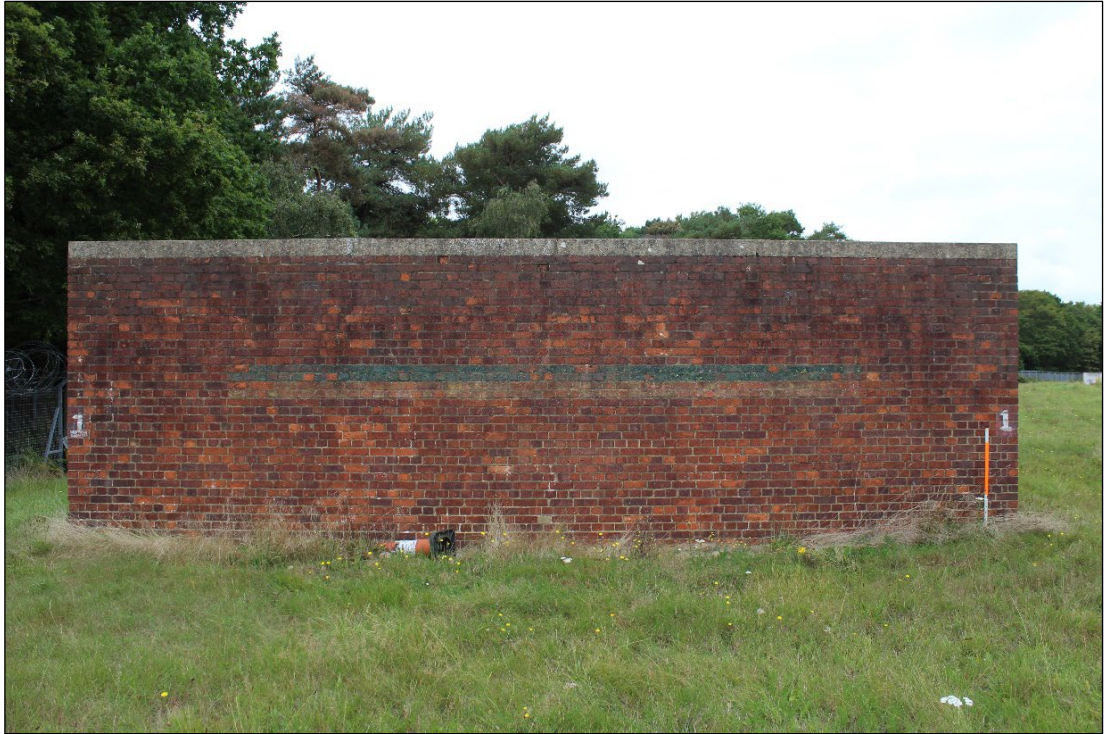
Photo 9: Apparatus Feature A1, viewed from the south
