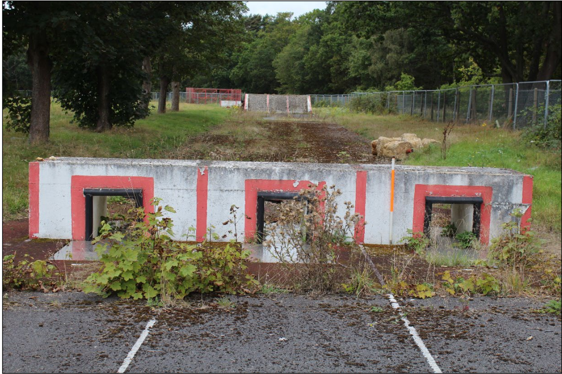
Photo 29: Apparatus Feature B1, viewed from the east
