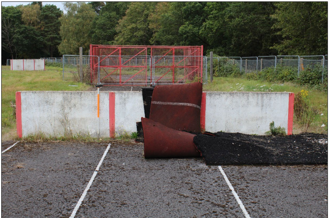
Photo 40: Apparatus Feature B4, viewed from the east
