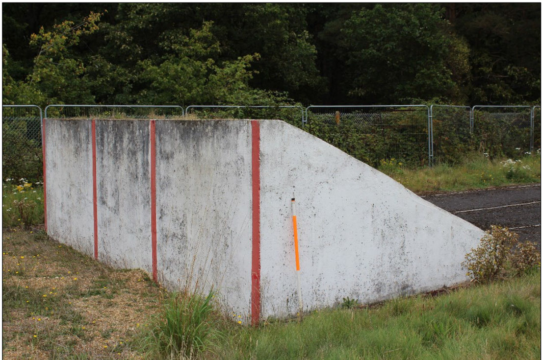
Photo 38: Apparatus Feature B3, viewed from the south-west
