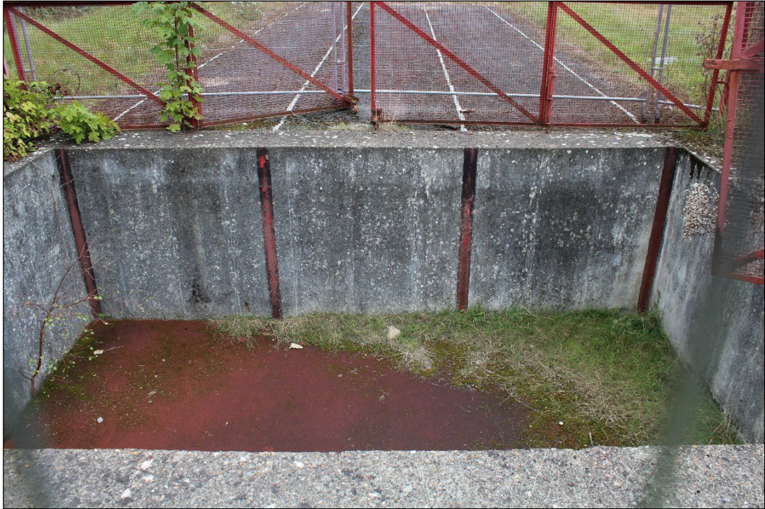
Photo 44: Apparatus Feature B5, viewed from the west
