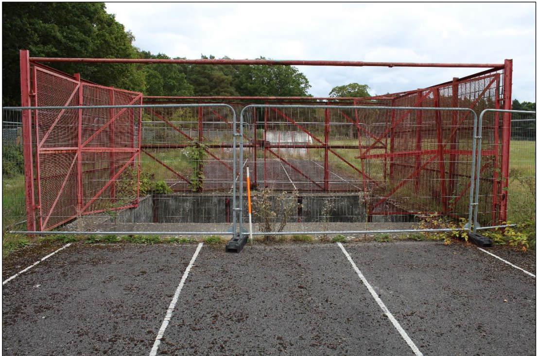
Photo 43: Apparatus Feature B5, viewed from the west
