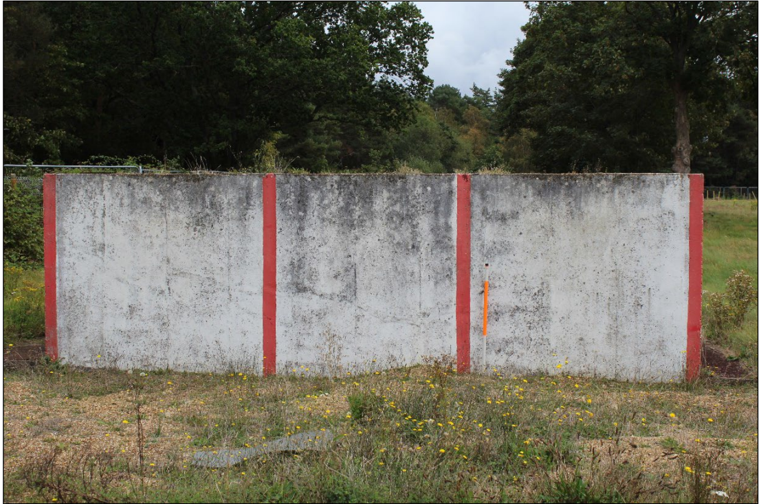
Photo 39: Apparatus Feature B3, viewed from the west.
