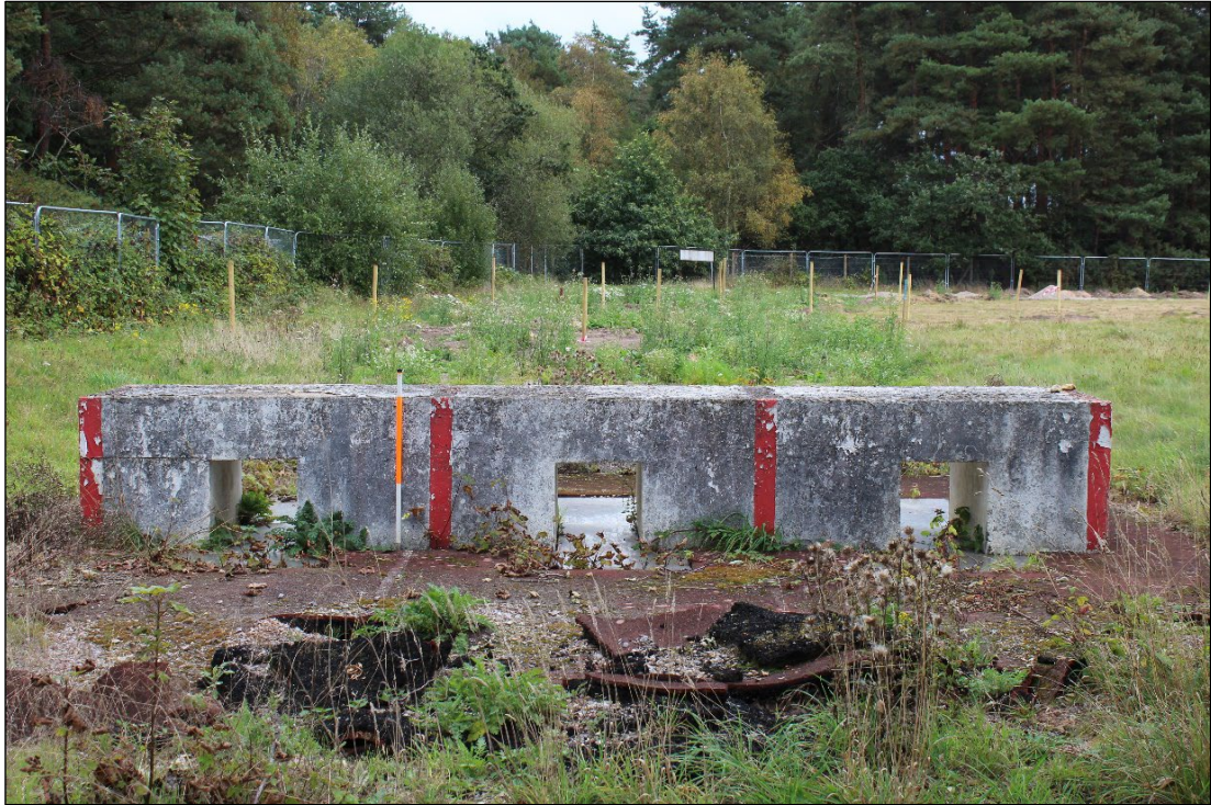
Photo 31: Apparatus Feature B1, viewed from the west
