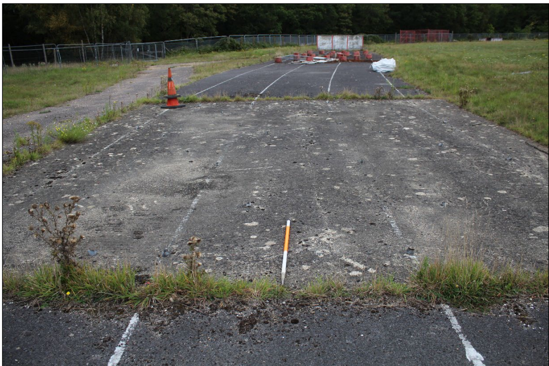
Photo 54: Apparatus Feature B9, viewed from the south-west
