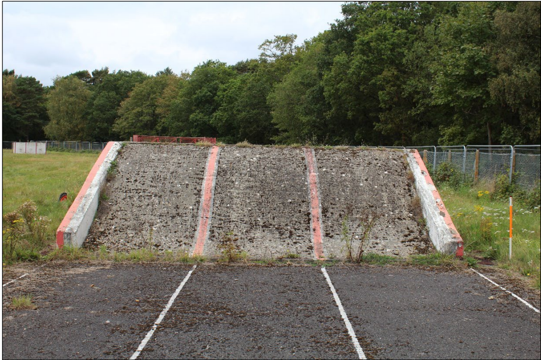
Photo 36: Apparatus Feature B3, viewed from the east
