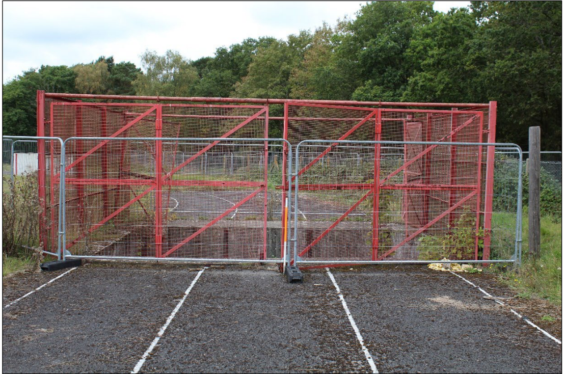
Photo 42: Apparatus Feature B5, viewed from the east
