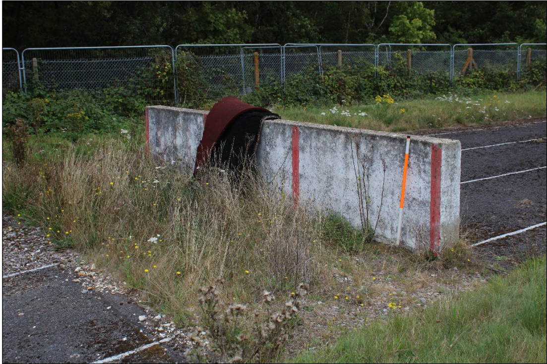
Photo 41: Apparatus Feature B4, viewed from the south-west
