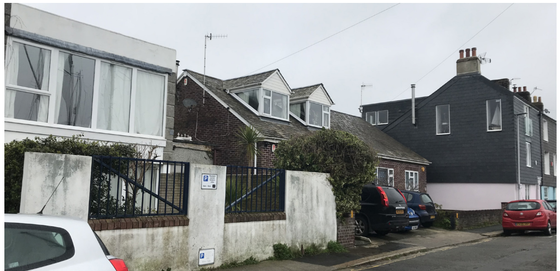
STREET VIEW LOOKING NORTH
