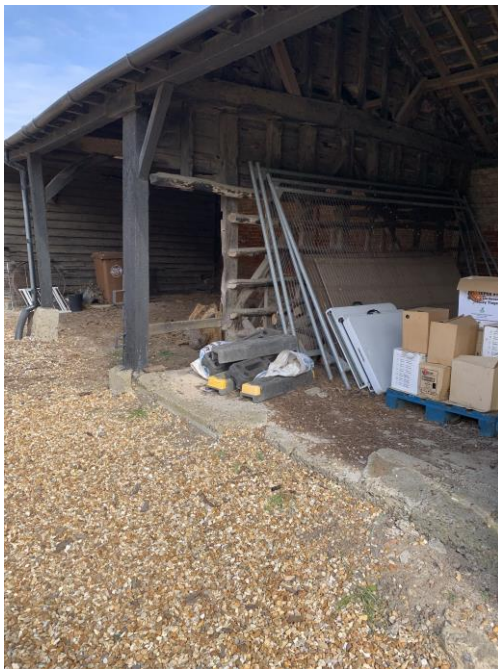
Site Photo 8: Interior view
