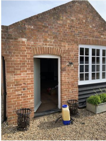
Site Photo 6: South Elevation view
