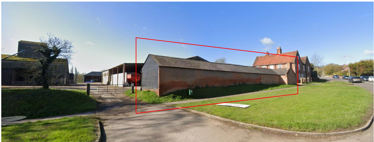
Site Photo 1: North and East Elevation
