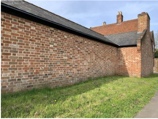
Site Photo 2: North Elevation
