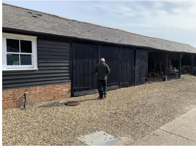
Site Photo 7: South Elevation view
