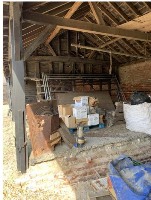
Site Photo 9: Interior view
