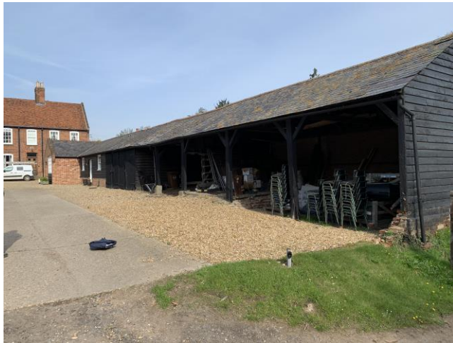
Site Photo 4: South Elevation
