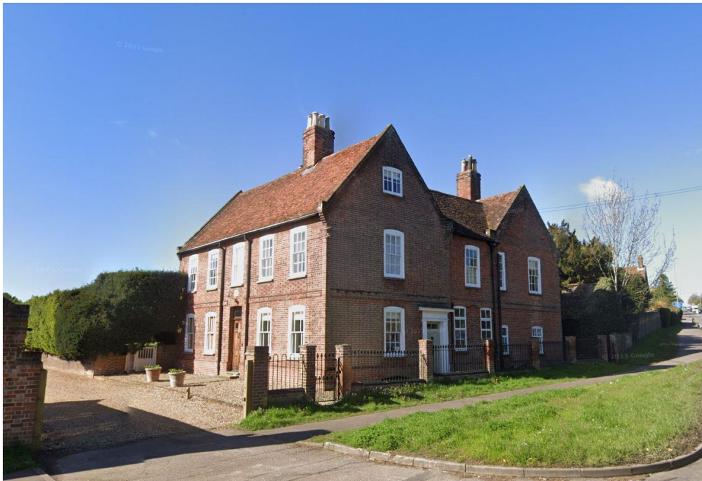
Site Photo 1: Front and Side Elevation
