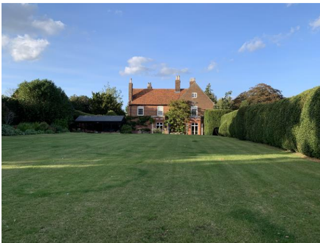
Site Photo 2: Rear Elevation
