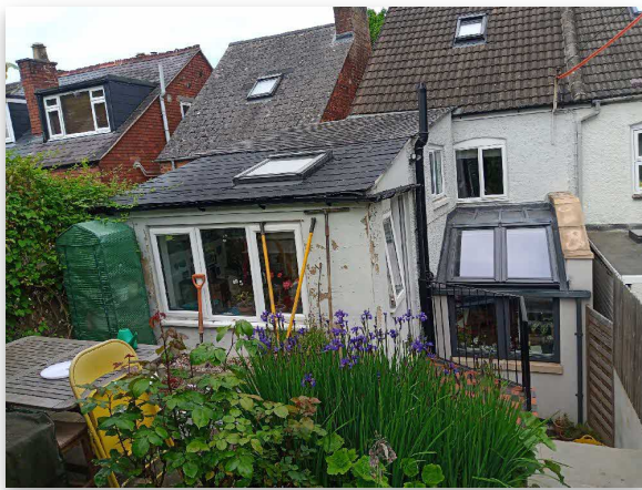
Fig 1.1: Trial Hole 1 Location
