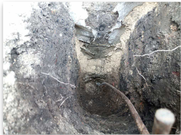
Fig 1.2: Trial Hole 1 Footing
