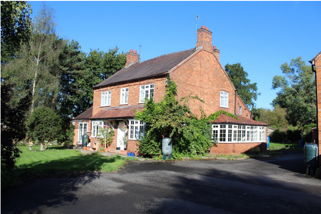
Image EDP A2.4: View from south-east toward Camp Farm farmhouse. Note the modern extensions, including bay windows on main elevation, and replacement uPVC door and windows.
