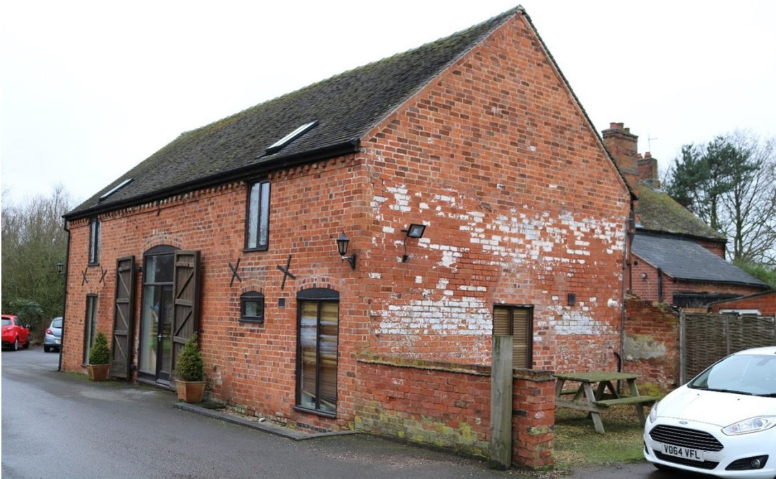
Image EDP A2.5: View from the north-east toward Camp Farm barn. Note the modern roof, windows and doors.
