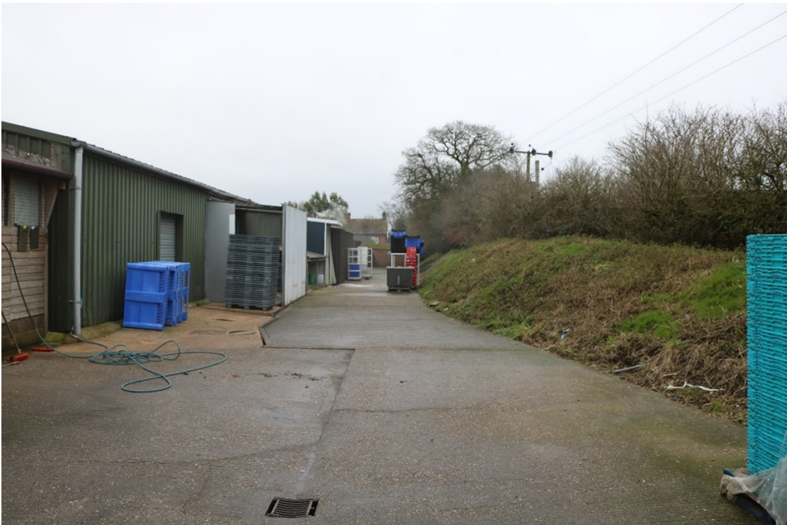
Image EDP A2.9: View southward, along the western edge of the Camp Farm light industrial complex. Note the earth bank to the right of the photograph, which provides evidence for the amount of earth movement during the construction of the hardstanding and modern buildings.
