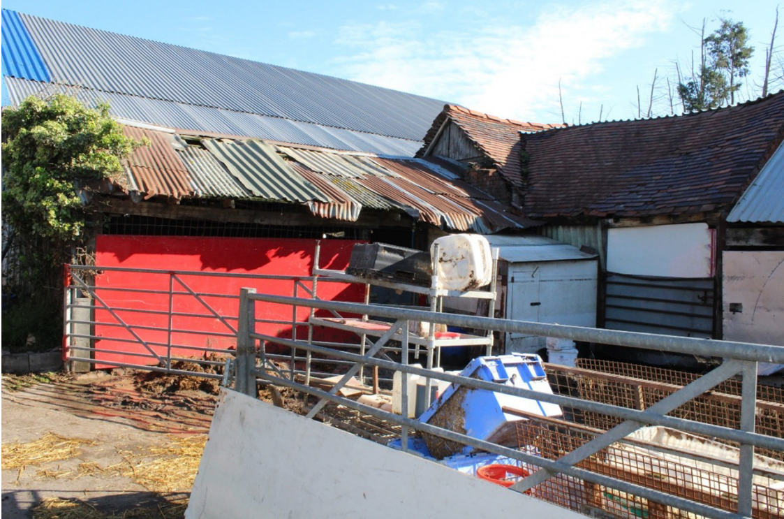
Image EDP A2.7: View from the south-west toward the L-shaped range at Southview Farm. Note that it is heavily altered, with the northern arm of the 'L' (on the left of the picture) surviving as a timber skeleton with a corrugated iron roof.
