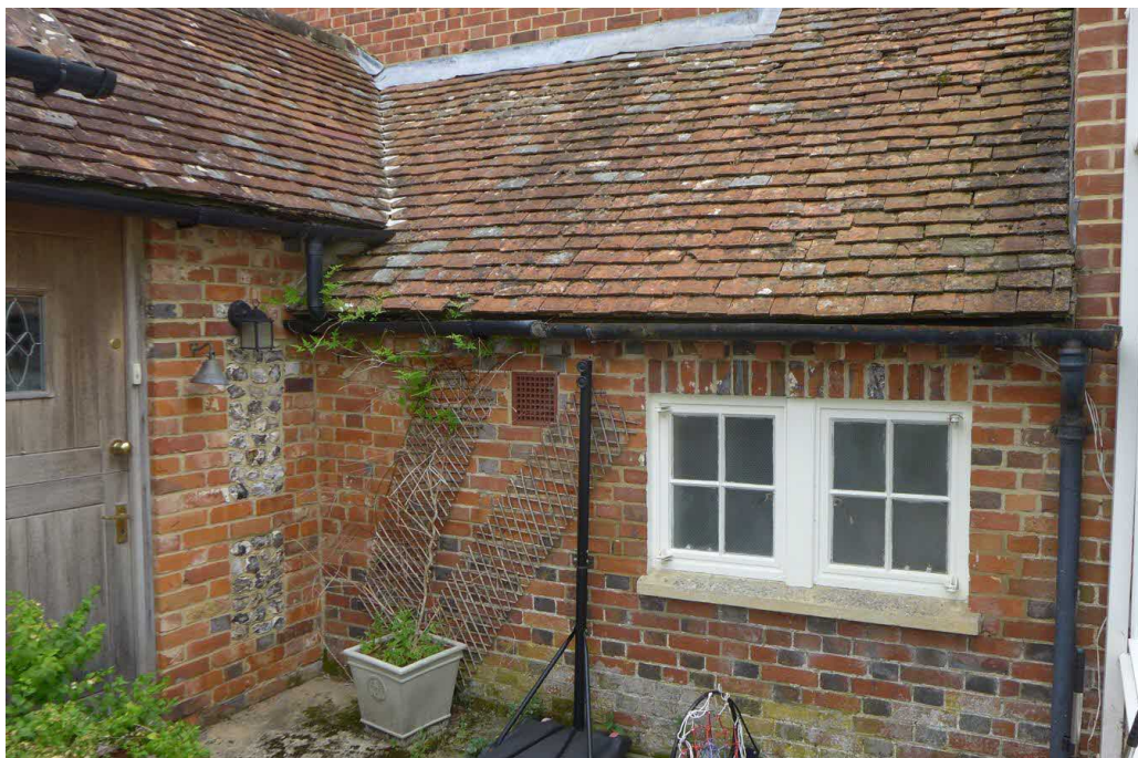
Pl.16: The north side of the Linking Range; note modern window, the use of cement mortar and plainer brick above 500mm and bonding in of the two sections on the left-hand side.
