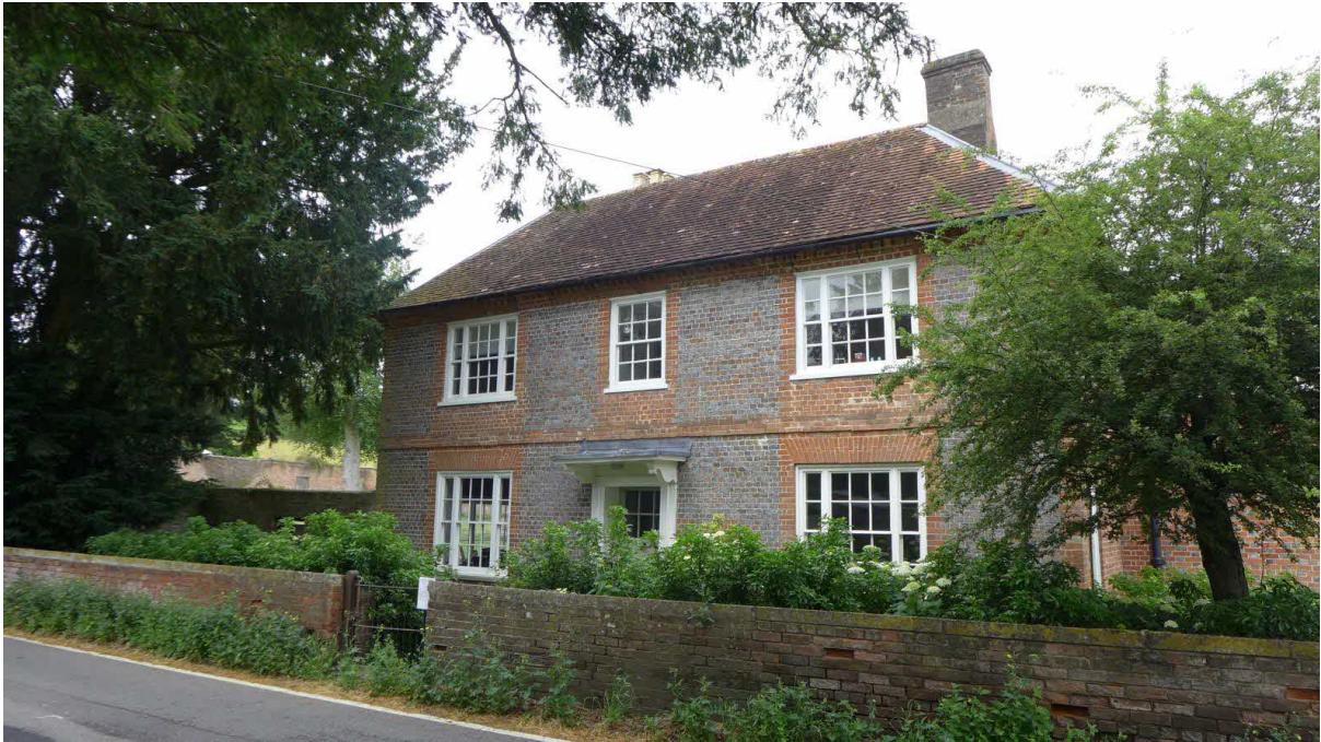
Pl.2: The front, or south, elevation of the Main House.
