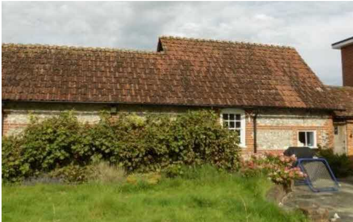
Image 1 – West facing elevation of the building
