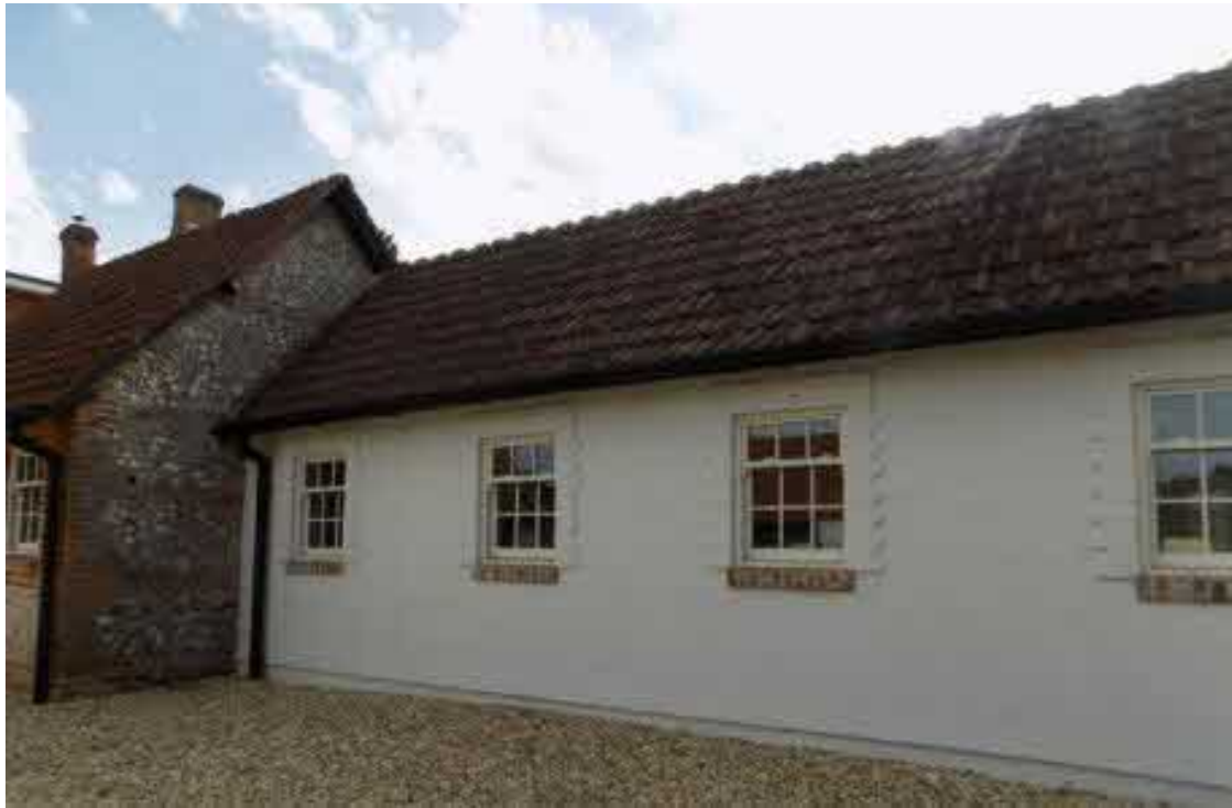
Image 3 – East facing elevation of the building
