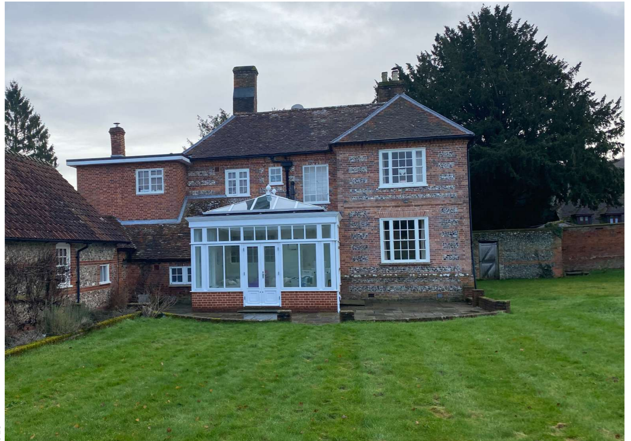
Rear elevation showing modern conservatory, lean-to abutting original building and linking range
