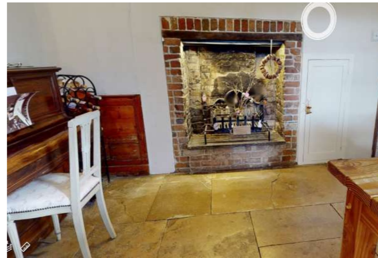
Original cooking range within existing dining room
